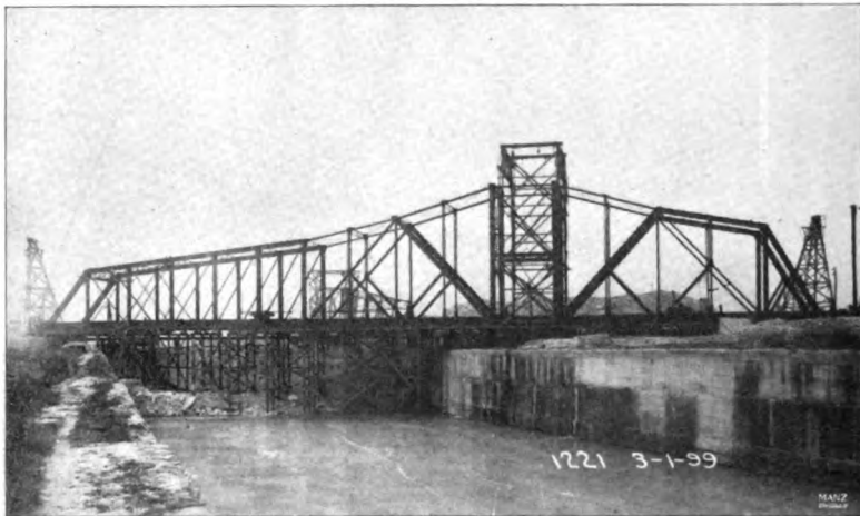
Fig. 12—Atchison, Topeka & Santa Fe Ry. Bridge, Section 8.
