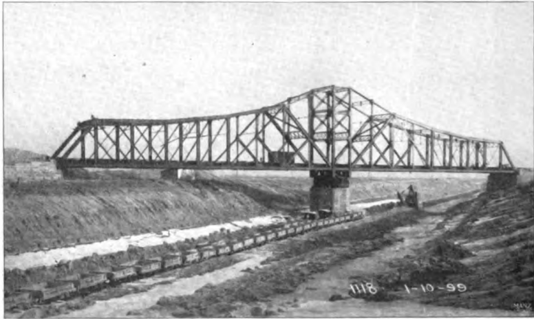
Fig. 7 Chicago, Madison & Northern R. R. Bridge.
