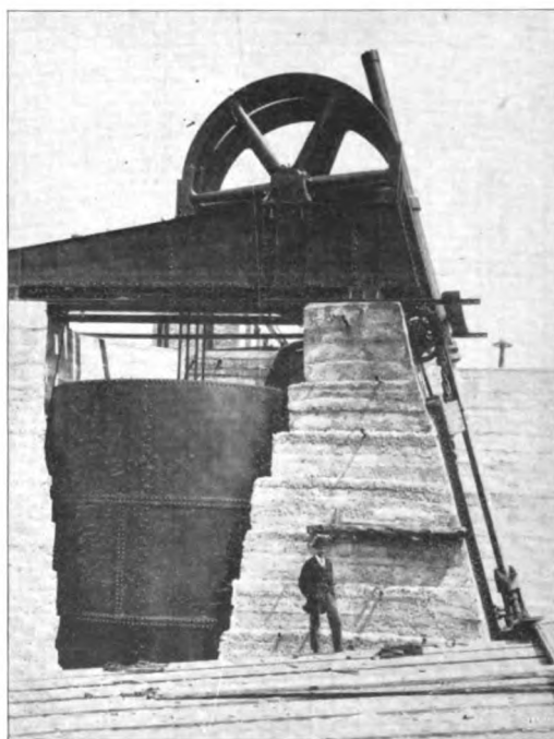
Fig. 17—Counter Weight Cylinder, Bear Trap Dam.
