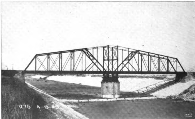
Fig. 10—Chicago Terminal Transfer R. R. Bridge.
