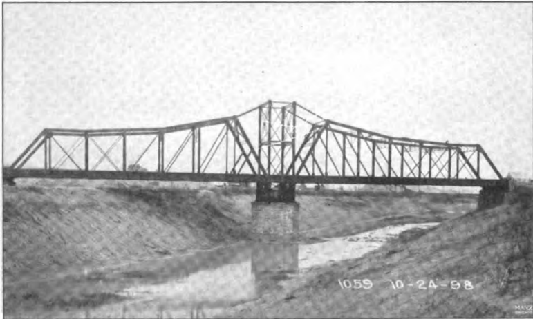
Fig. 8—Atchison, Topeka & Santa Fe Ry. Bridge, Section G.
