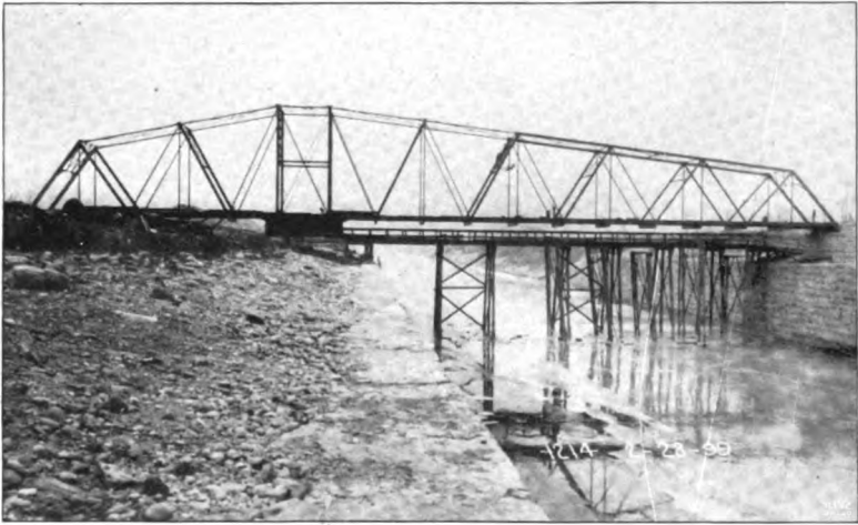
Fig. 11—Willow Springs Highway Bridge.
