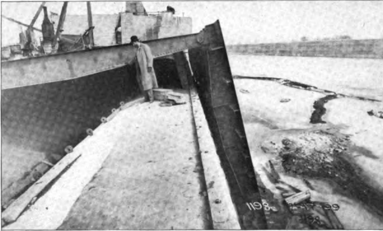
Fig. 18—Construction View, Bear Trap Dam.
