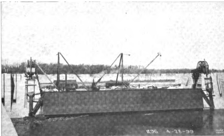
Fig. 19—Front View, Bear Trap Dam.
