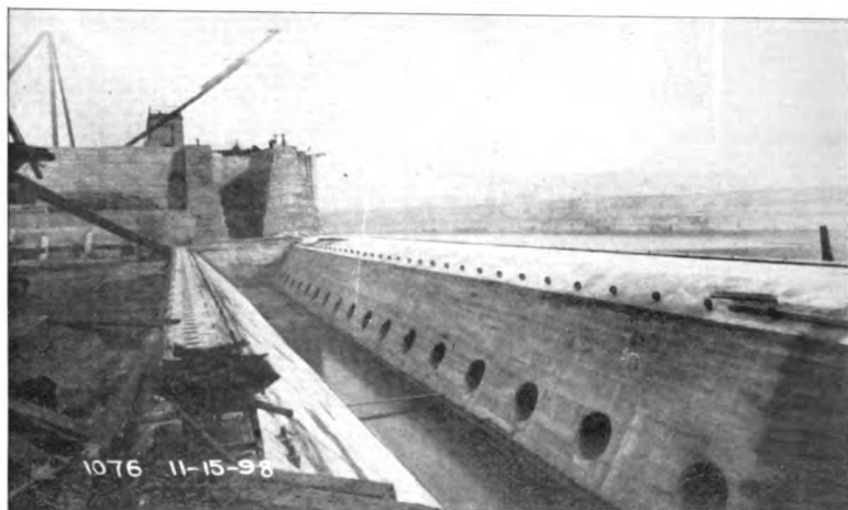
Fig. 16—Foundation, Masonry and Conduit, Bear Trap Dam.
