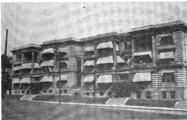
Lafayette and Cambridge Apartments, McKee Place, erected 1902, equipped with wrought iron pipe. Most of the hot water mains were replaced in 1917, after 14 years' service. Record No. 42, Wrought Iron Installations, page 17.
