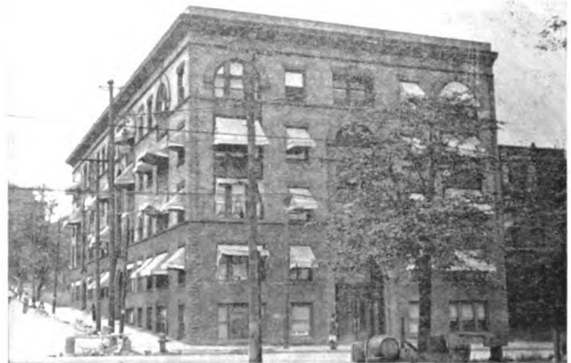
Oakland Apartments, Halket and Forbes Streets, erected in 1902, and equipped with wrought iron pipe, all of which is still in good condition, excepting the hot water mains which now need replacement after 15 years' service. See record No. 55, Wrought Iron Installations, page 18.
