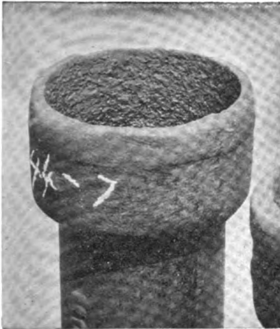
Fig. 2—Cast Iron. Showing Typical Corrosion Resulting in Even Pock-marking or Shallow Pitting.
