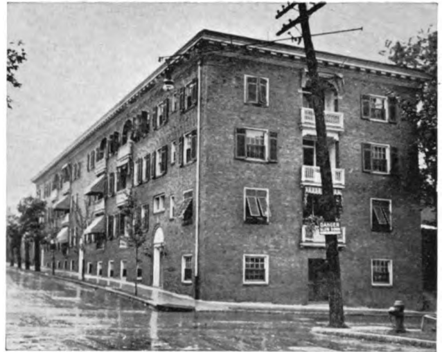
Negley Apartments, erected 1909. Hot water mains of steel, largely replaced between 1911 and 1914. Trouble with rusty water. See record No. 1, page 15.
