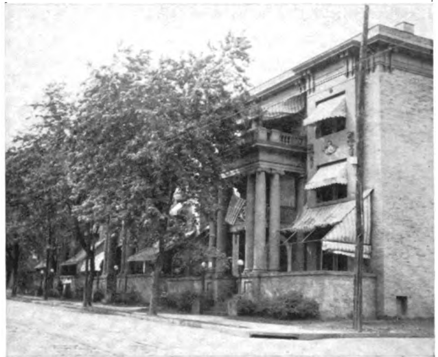
The Lexington, Argyle, and Drexel Apartments, erected 1909. Equipped with steel pipe. Life of hot water mains, 7 or 8 years. See records Nos. 13, 14 and 15, page 15.
