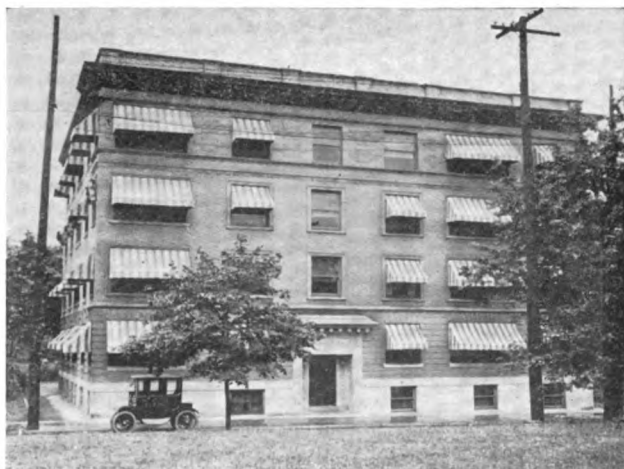
D'Arlington Apartments, erected 1909, equipped with brass pipe. The hot water lines are badly corroded and pitted after 8 years' service. Record No. 7, Brass Installations, page 13.
