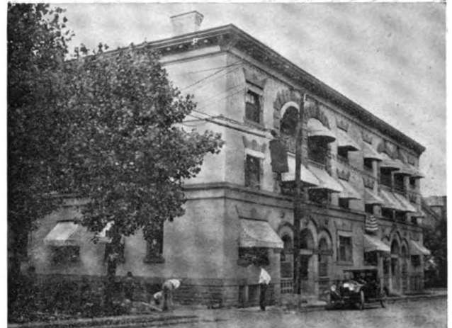
The Howe and Kent Apartments, erected 1907. The hot water mains are of brass and already show pitting. See records on brass piping, page 14.
