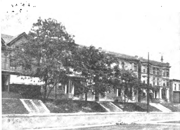
Yellow Brick Apartments, erected 1902. Equipped with wrought iron pipe. Hot water mains needing replacement after 14 years' service, See records Nos. 43 and 44, page 17.
