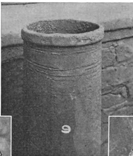
No. 9 35 Years Old Cast Iron Covered by Lead Coping. Gaff Building.
