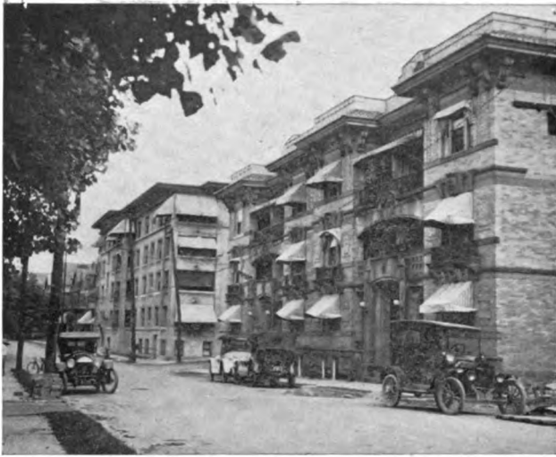
St. Regis, Chesapeake, and Chamberlin Apartments, erected 1908. Equipped with steel pipe. Most of the hot water mains have already been replaced. See records Nos. 17, 18 and 19, page 15.
