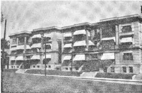
Lafayette and Cambridge Apartments, McKee Place, Pittsburgh, Pa., erected 1902. Wrought iron pipe in hot water mains had a life of 14 years in these apartments—twice the average life of steel pipe in the same service. Byers Bulletin No. 30, containing the results of an investigation conducted to determine the relative life of iron and steel pipe in hot and cold water lines in buildings, will be sent on request.
