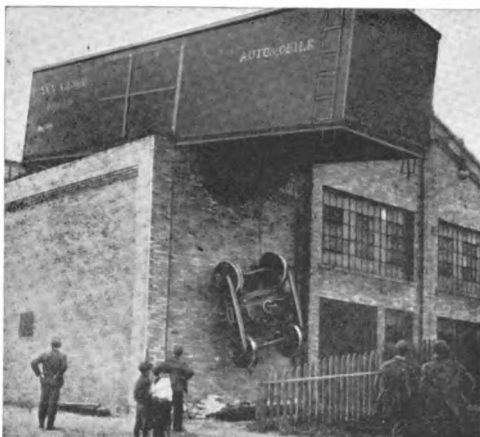
At North Rochester, Pa., a freight car recently ran off an elevated siding and lodged on factory roof as shown in picture. The front truck was torn loose but stopped in mid-air, suspended by the genuine wrought iron brake rod, only \frac{3}{4} in. in diameter; a striking illustration of the toughness and strength of genuine wrought iron. (Compare with statement of Wallace G. Imhoff, Consulting Engineer, page 4.)
