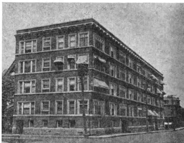
The Netherlands Apartments, Summerlea and Elwood, erected 1911, equipped with steel pipe. The hot water soon became so rusty that filters were installed in 1916. These filters, however, have not eliminated the rust from the water. See record No. 20 on page 15 and also paragraph on "Rusty Water" on page 7.
