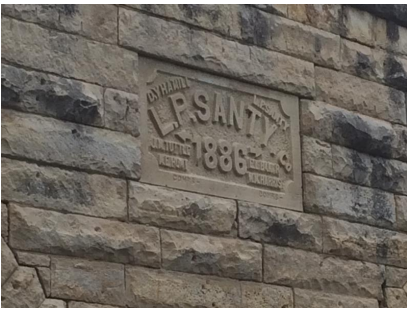
Clements Stone Arch Bridge
