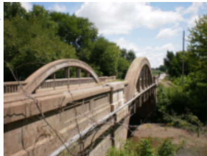
Rock Creek Bridge. View toward east. KRingler. 7-30-09
