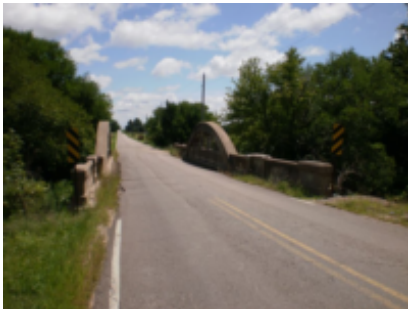
Rock Creek Bridge. View toward east. KRingler. 7-30-09
