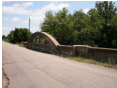
Rock Creek Bridge. View toward east. KRingler. 7-30-09
