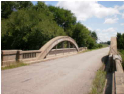
Rock Creek Bridge. View toward east. KRingler. 7-30-09
