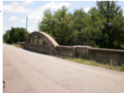
Rock Creek Bridge. View toward east. KRingler. 7-30-09
