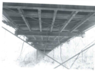
Big Slough Creek Truss Bridge. Substructure. 04/10/1981.
