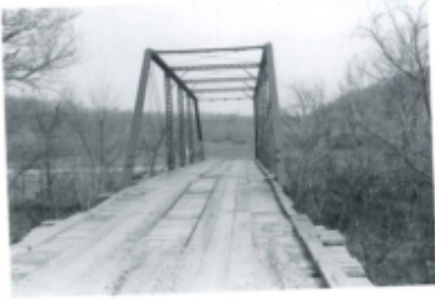
Big Slough Creek Truss Bridge. Looking east. 04/10/1981.
