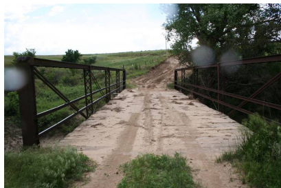
Sand Creek Truss Leg Bedstead Bridge. 2013.
