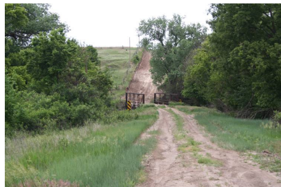
Sand Creek Truss Leg Bedstead Bridge. 2013.
