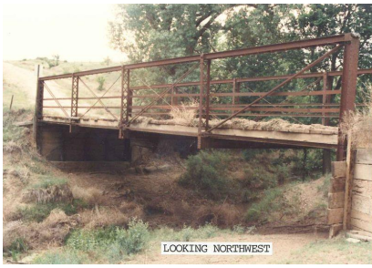
Sand Creek Truss Leg Bedstead Bridge. 1989.
