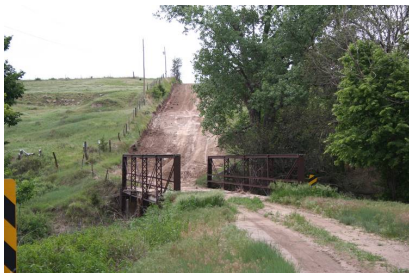
Sand Creek Truss Leg Bedstead Bridge. 2013.
