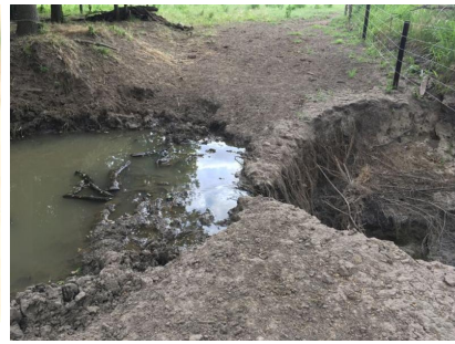
Sand Creek Truss Leg Bedstead Bridge. Lenora vicinity. Proposed location, facing E. July 2017.
