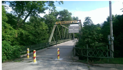
Lindsborg Truss bridge on South 1st street; photo July 2 2016 by Wallen
