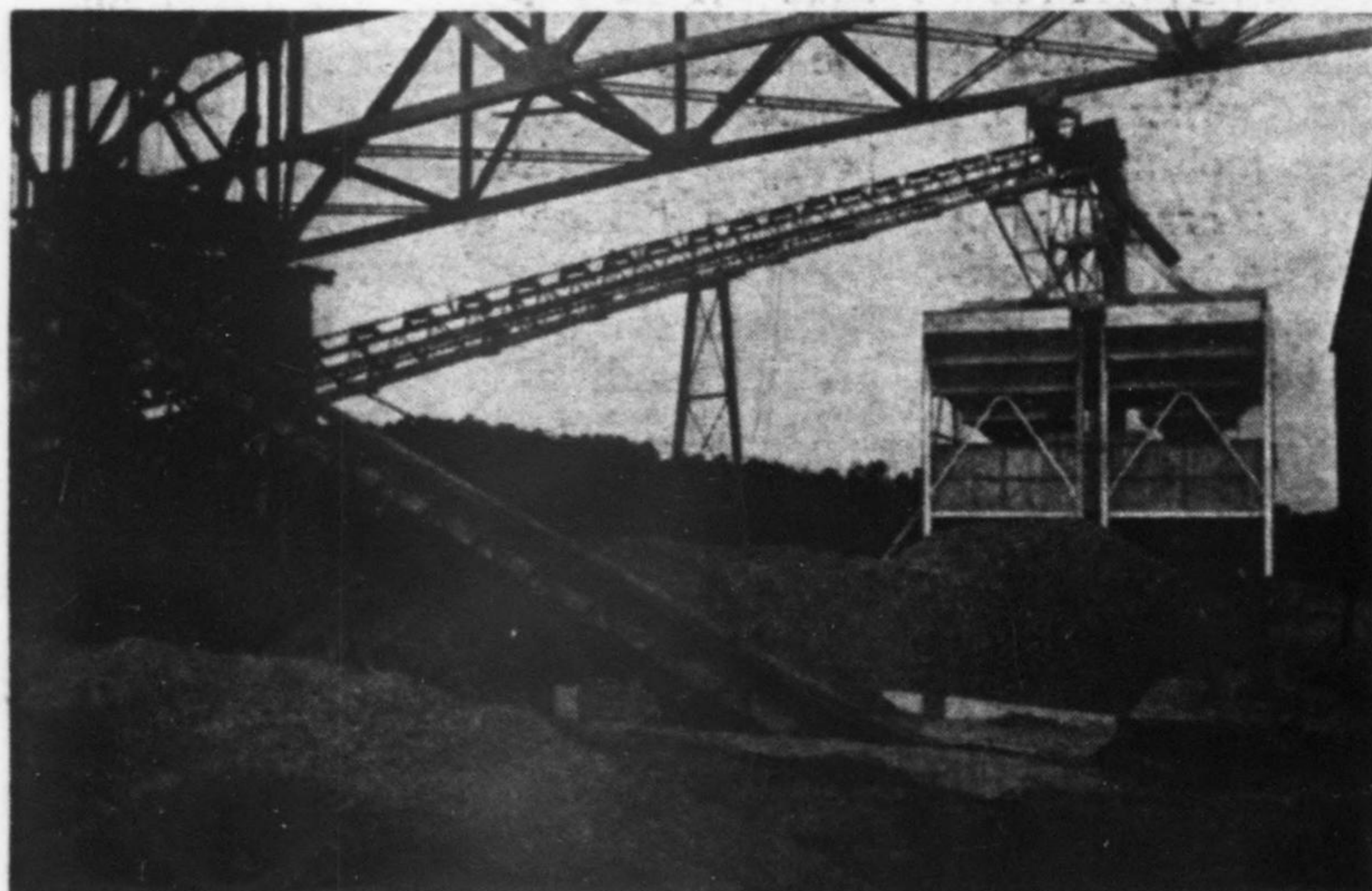
FIG. 4—TWO VIEWS of the batching plant, whose layout is shown in Fig. 3. Left: aggregate-handling conveyors with railway car at extreme right and bridge superstructure overhead. Right: cement end of plant with bulk-cement cars on left-hand track.
