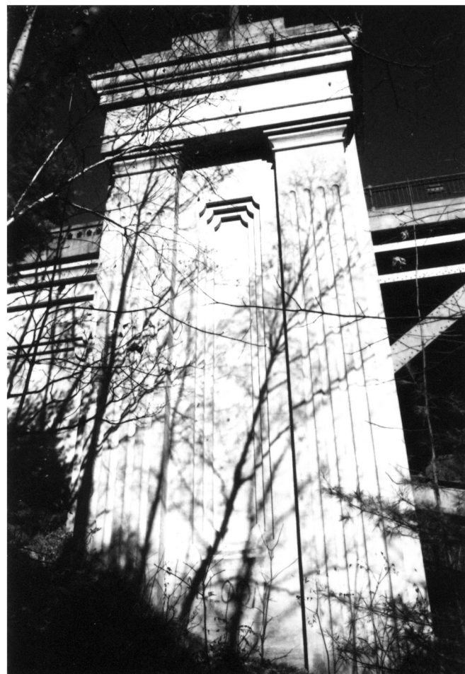
W abutment, S pylon, from S
