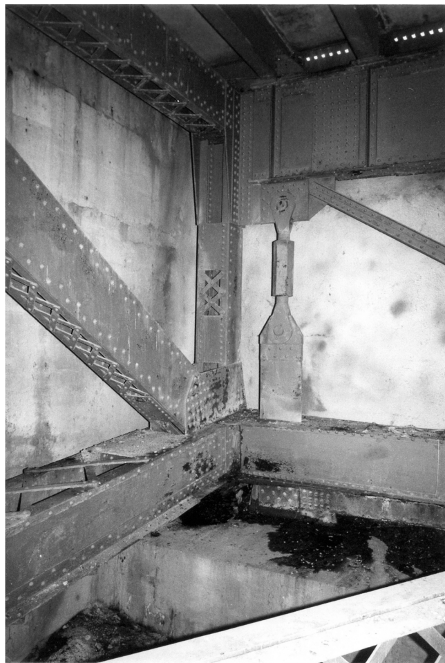
Bearing and anchor at western end of southern line of arches
