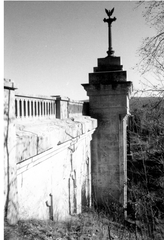
South face, west abutment, from West
