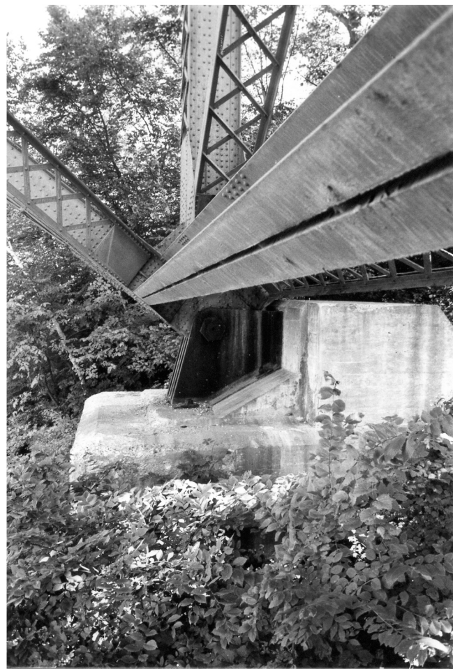
Northern arch, eastern hinge and abut., from SW
