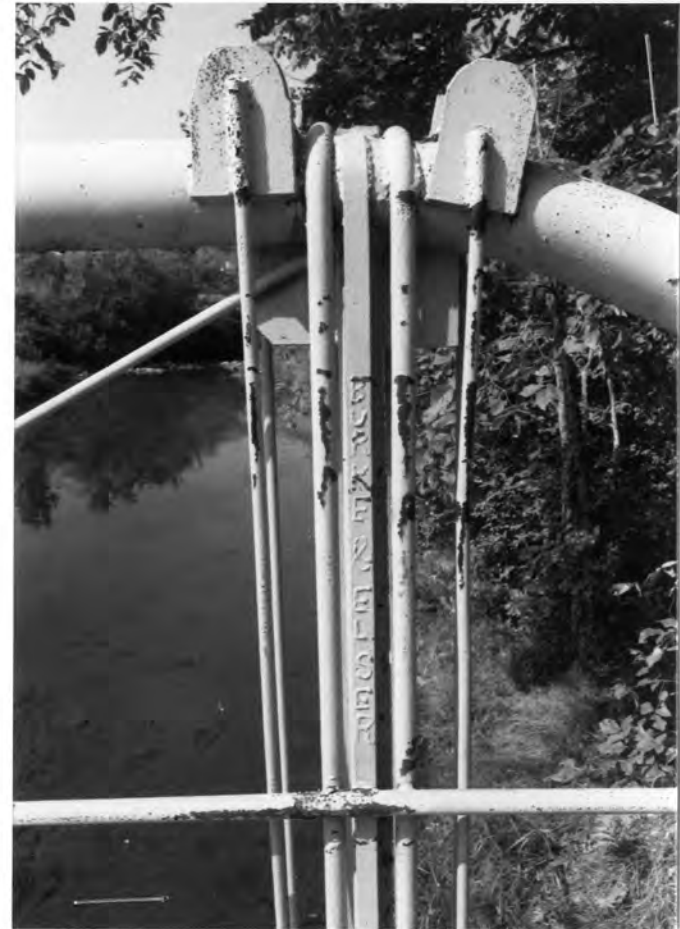
W TRUSS, NORTHERN UPPER PANEL POINT, FROM E
