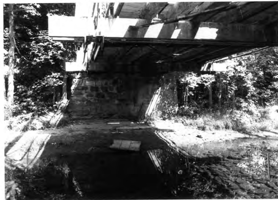
N ABUTMENT FROM S
