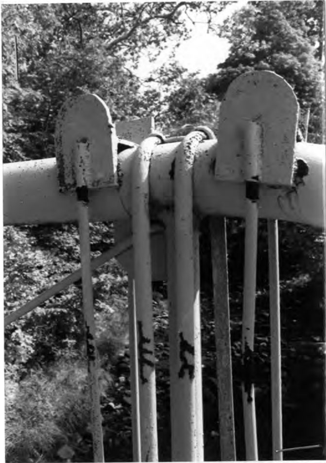
EAST TRUSS, SOUTHERN UPPER PANEL POINT, FROM SW
