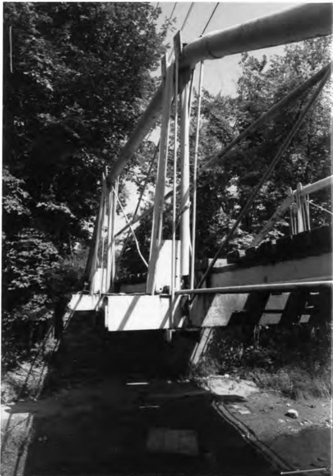
W TRUSS FROM S
