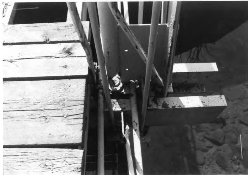
W truss, Sern lower panel point, from N
