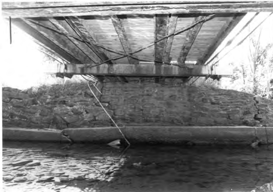
S ABUTMENT FROM N
