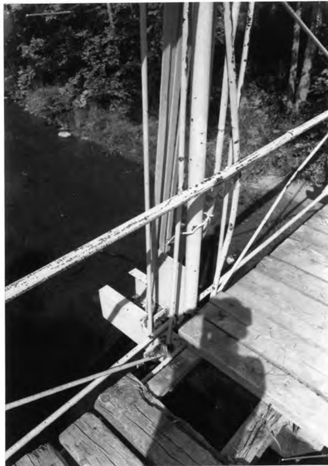
W TRUSS, SOUTHERN LOWER PANEL POINT, FROM SE
