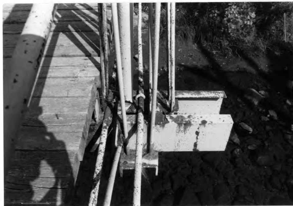
E Truss, Sern lower panel point, from S.
