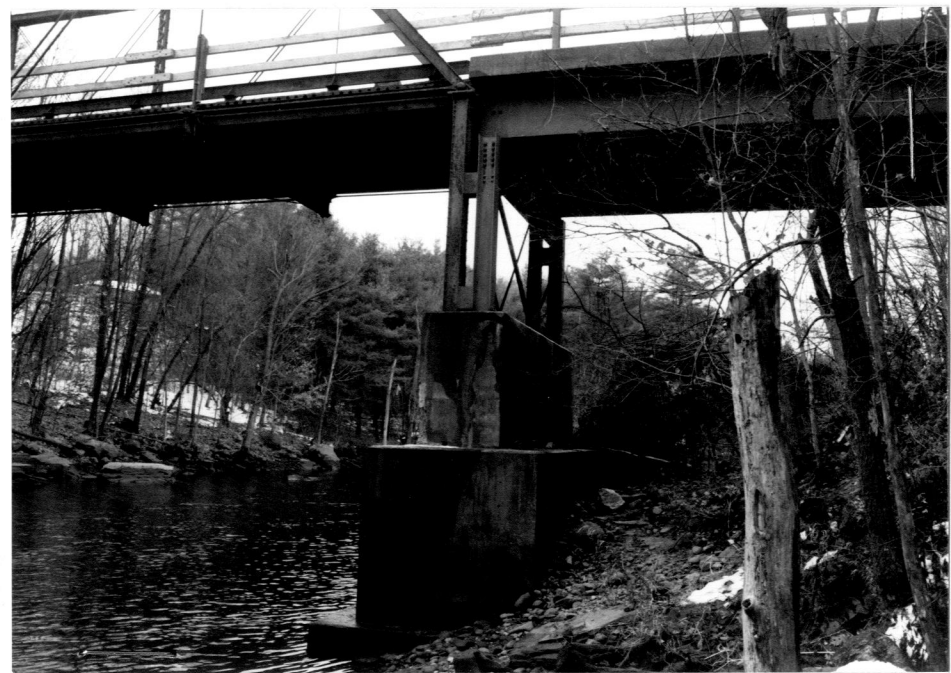
PIER, FROM N (11-17-87)
