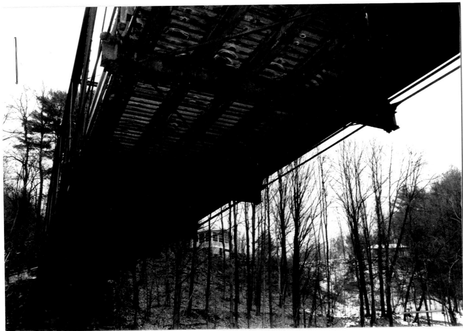
FROM N END OF PIER, LOOKING E (11-17-87)
