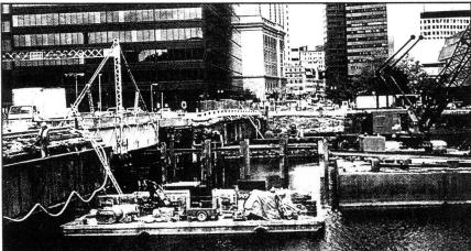
The Summer Street Bridge was kept open to both pedestrian and vehicular traffic during renovation, all of which was staged from barges.
