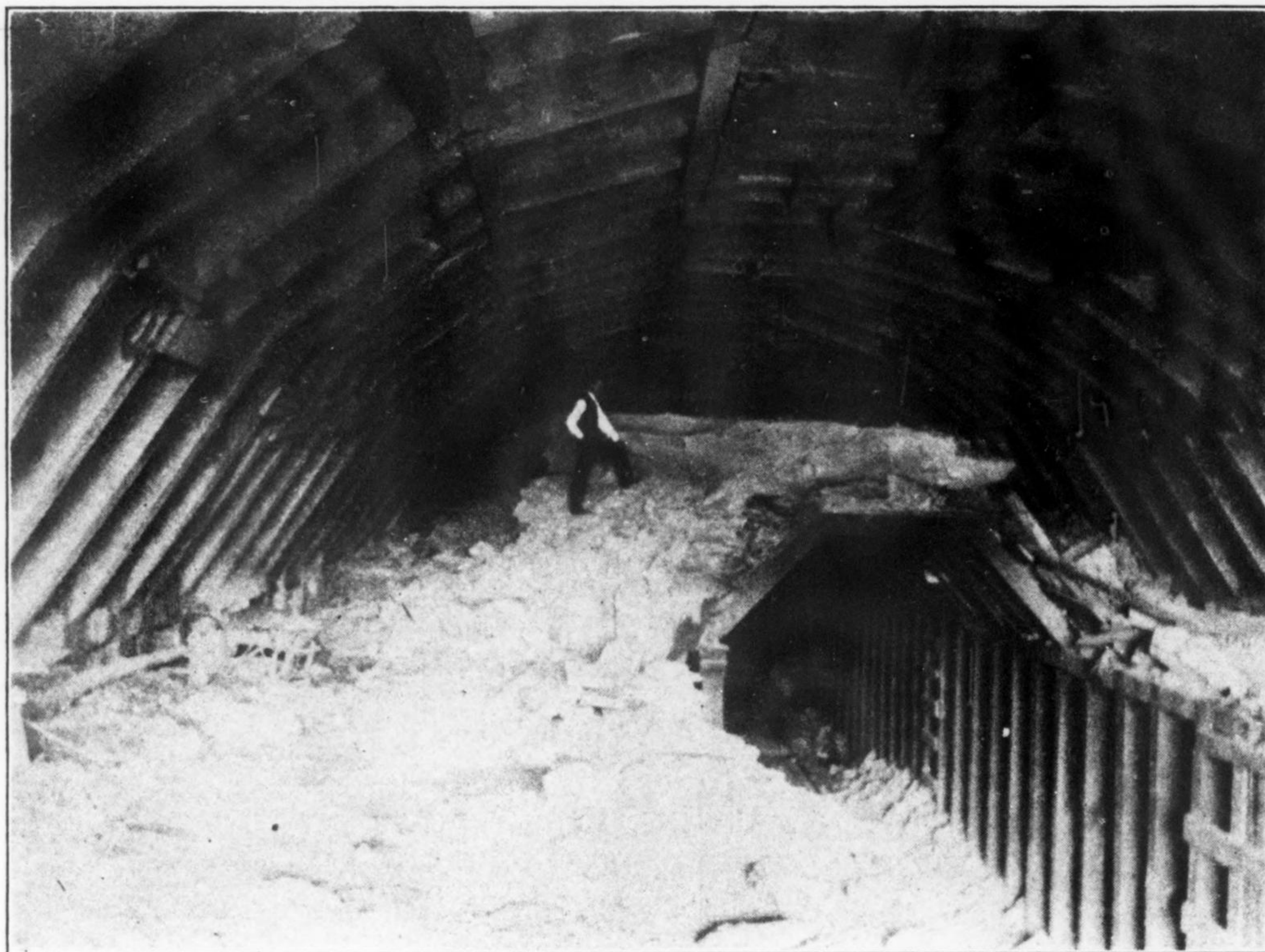
Double-Tracking the Barton Tunnel—C. L. & W.
