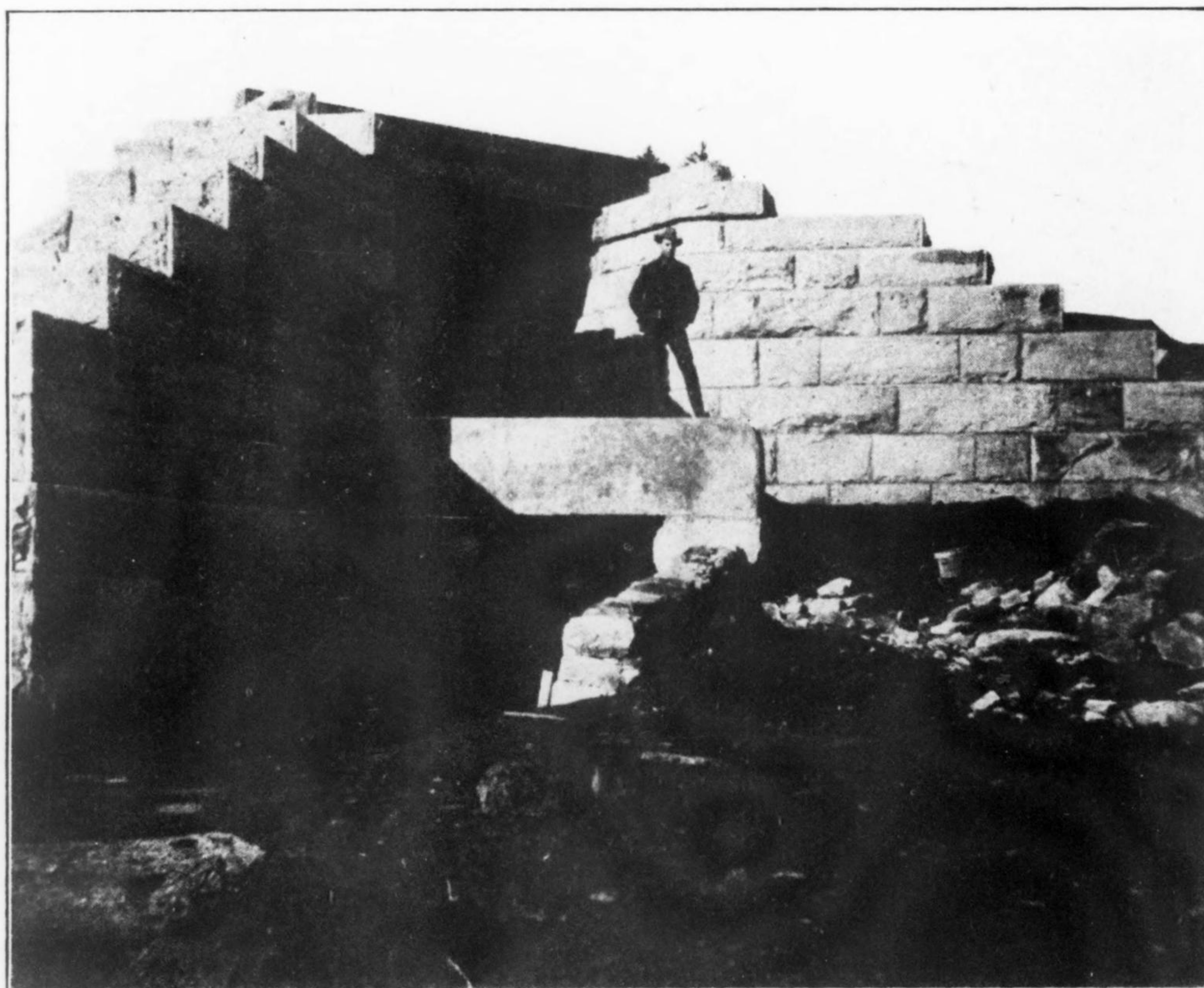
Walker's Undercrossing—C. L. & W.
