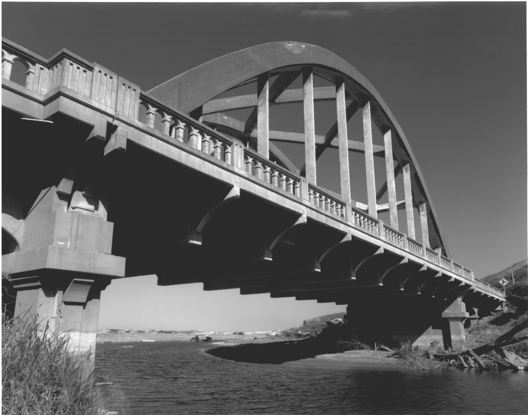
BIG CREEK BRIDGE, HECETA HEAD VICINITY, OREGON #2
