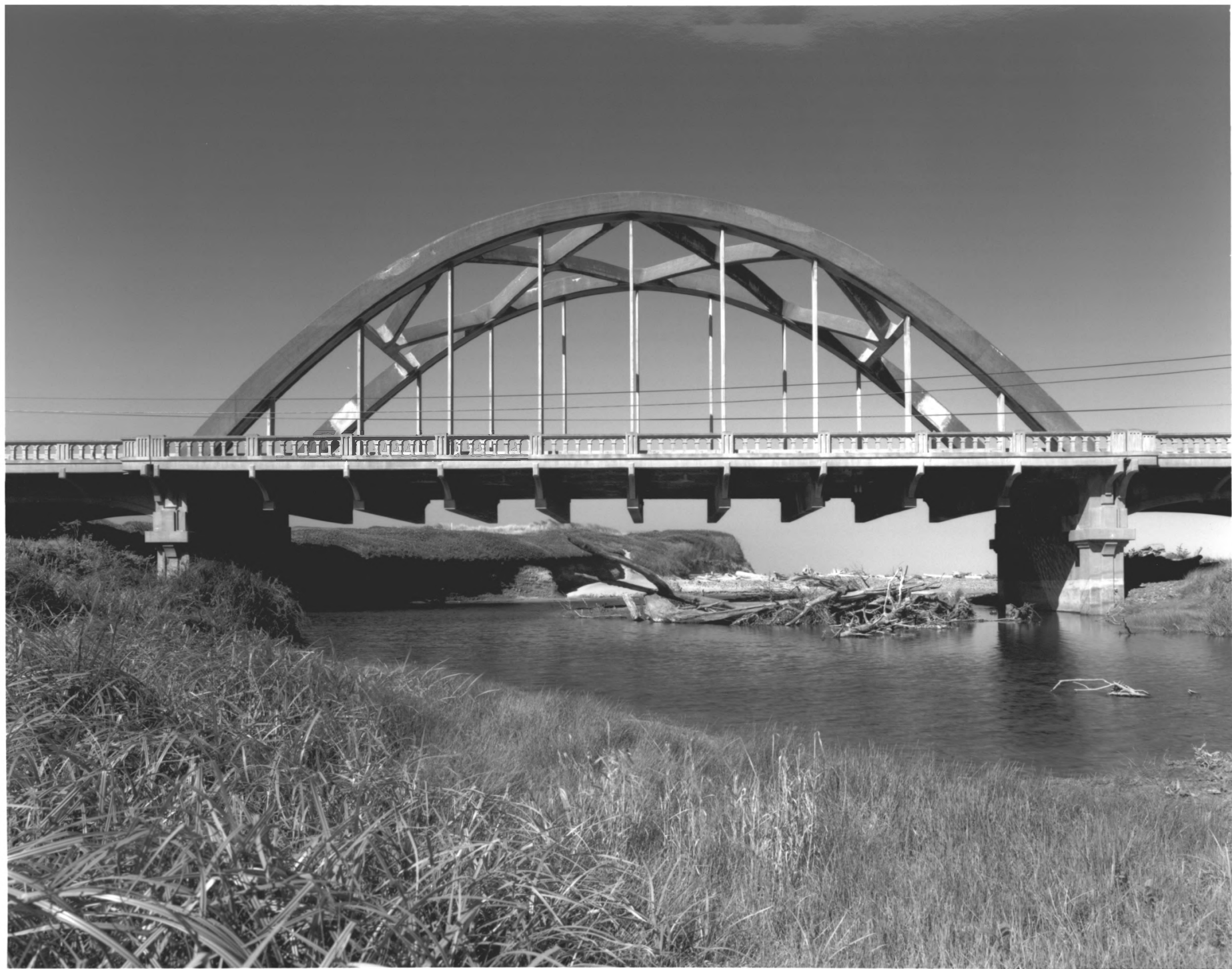
BIG CREEK BRIDGE, HERETA HEAD VICINITY, OREGON #3
