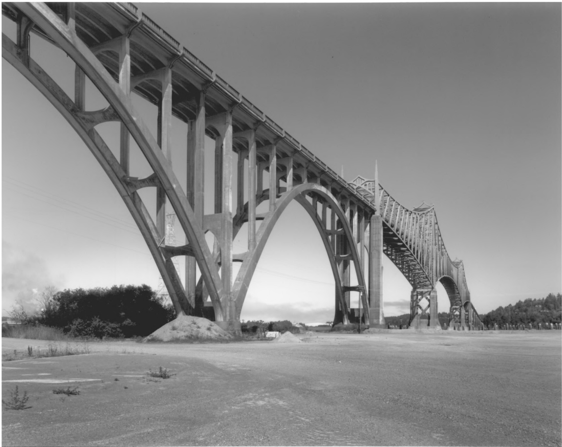
COOS BAY BRIDGE, COOS BAY, OREGON
