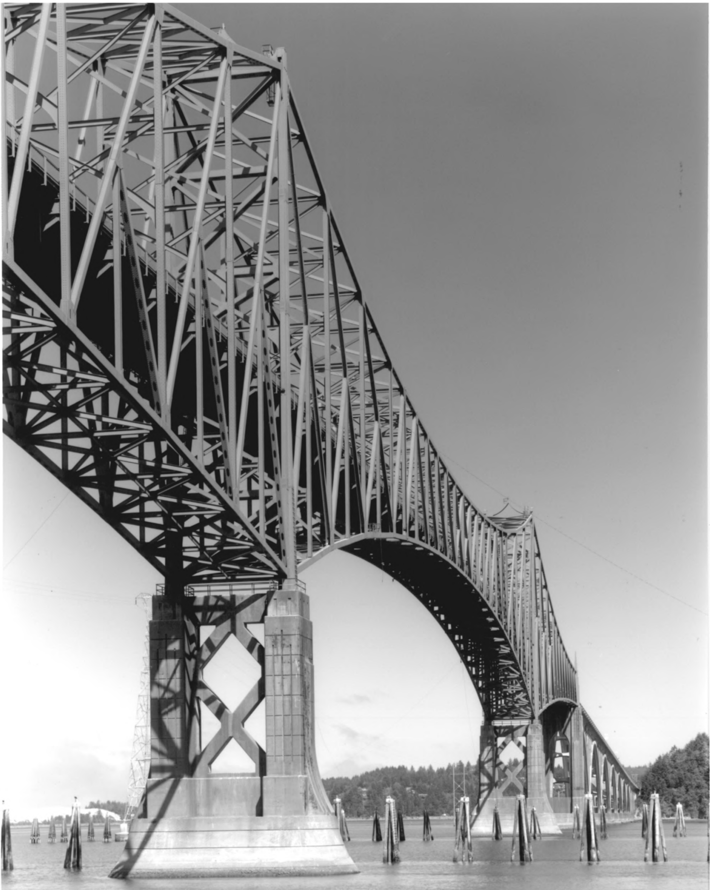
COOS BAY BRIDGE, COOS BAY, OREGON #8
