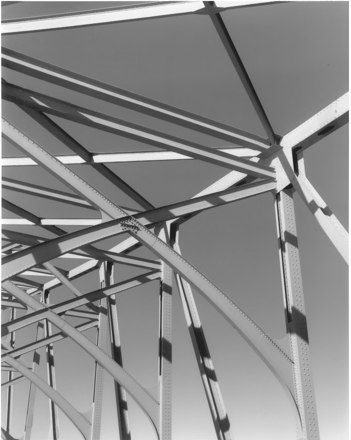
COOS BAY BRIDGE, COOS BAY, OREGON # 11
