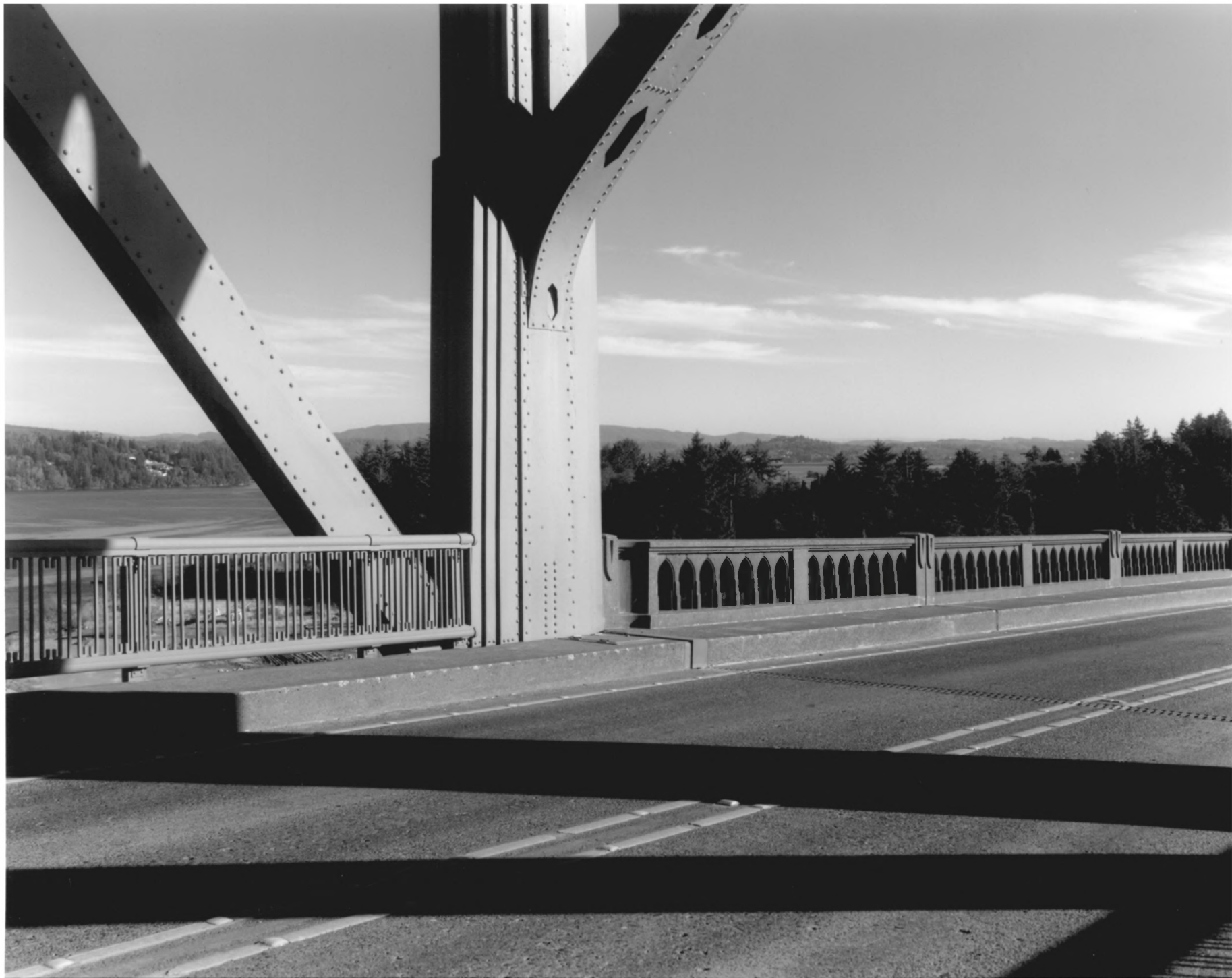
COOS BAY BRIDGE, COOS BAY, OREGON #10
