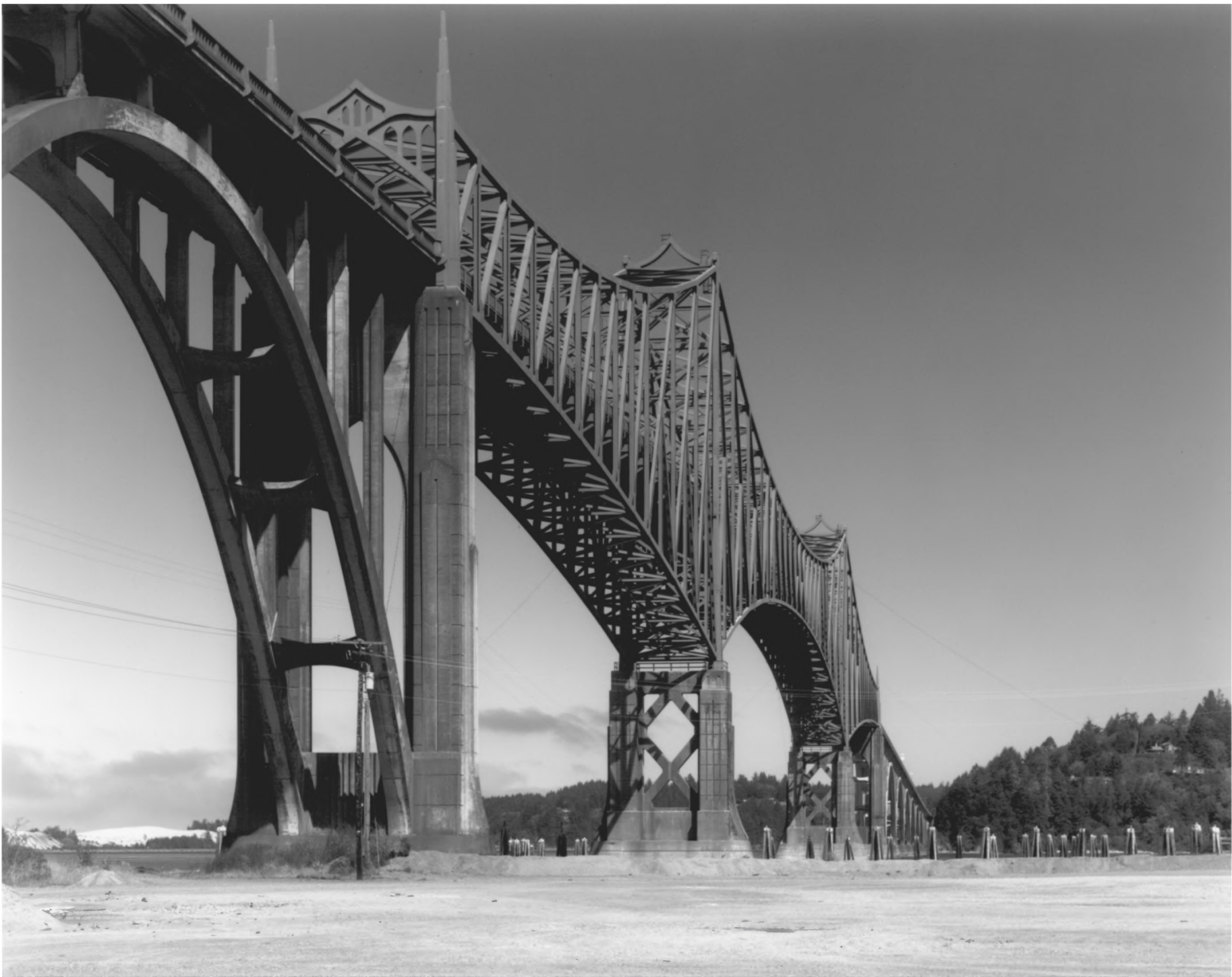
COOS BAY BRIDGE, COOS BAY, OREGON
