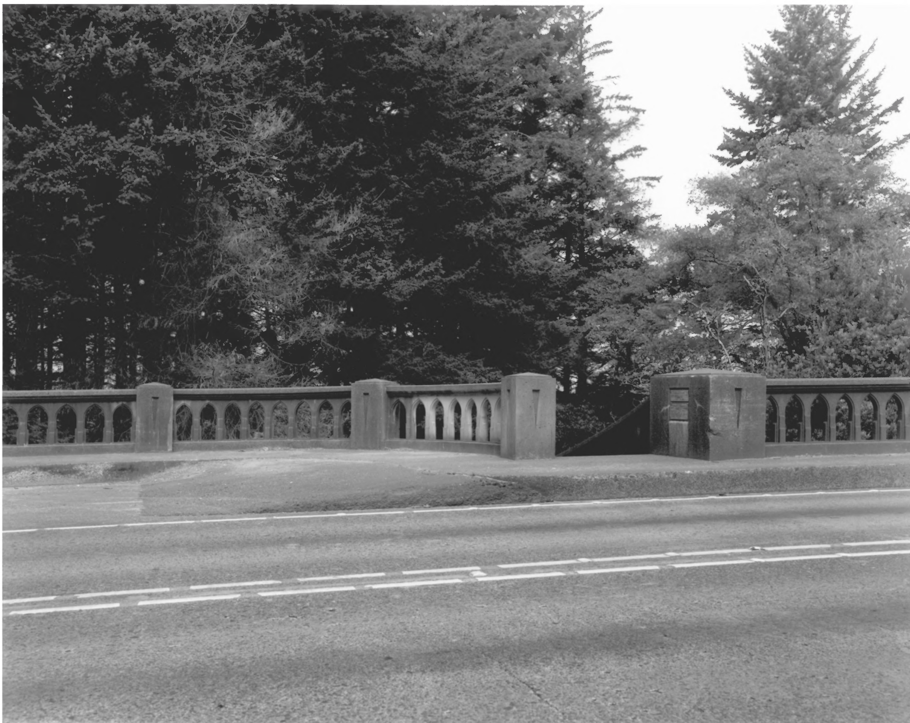
COOS BAY BRIDGE, COOS BAY, OREGON
