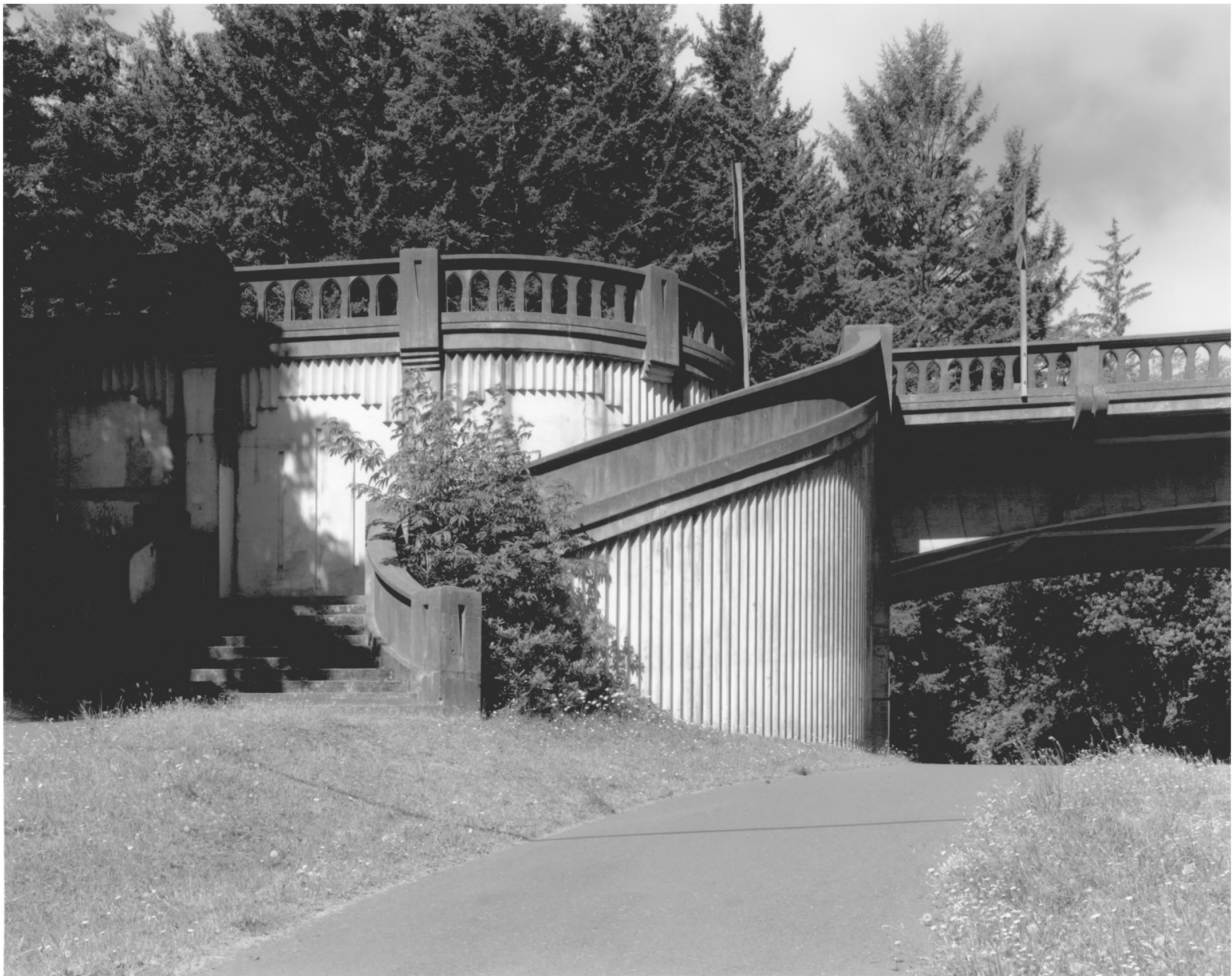
COOS BAY BRIDGE, COOS BAY, OREGON #12.
