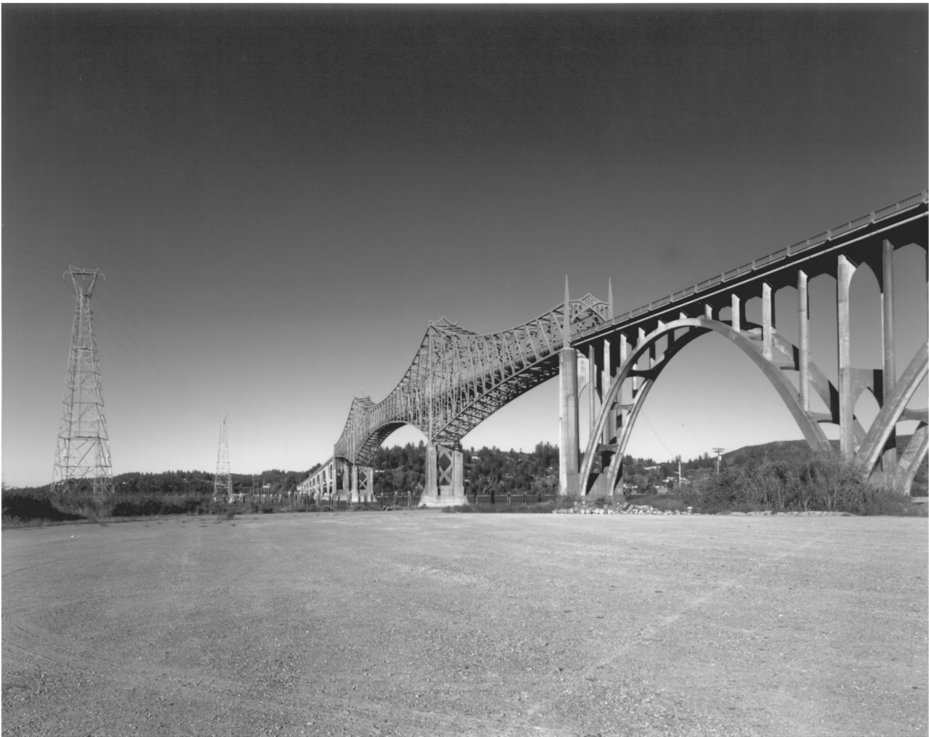
COOS BAY BRIDGE, COOS BAY, OREGON
