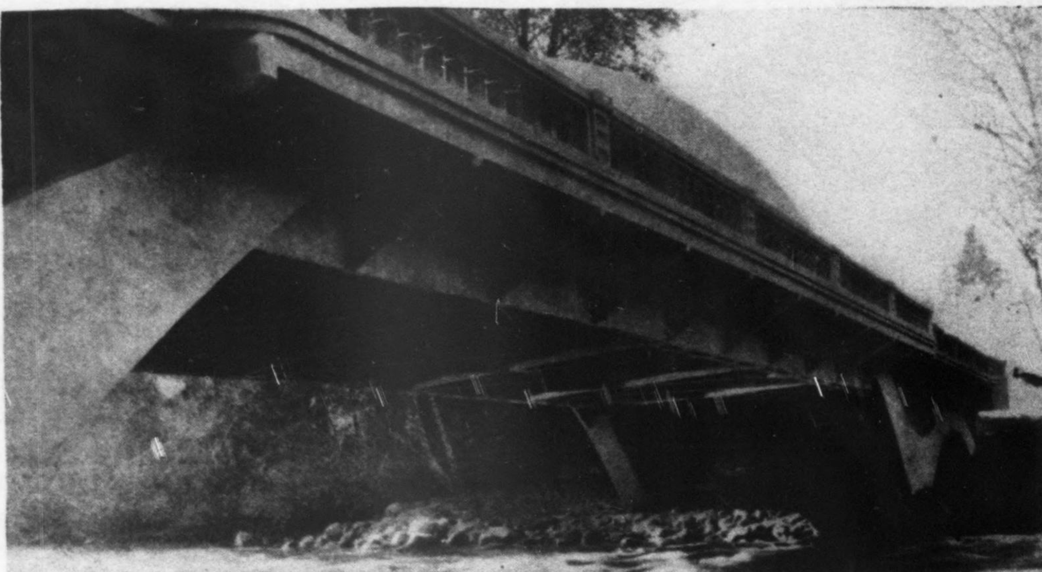
Fig. 4 (above)—Old suspension bridge, replaced by new arch, was utilized in erecting the new steelwork for the Oregon City Bridge in 1922.
