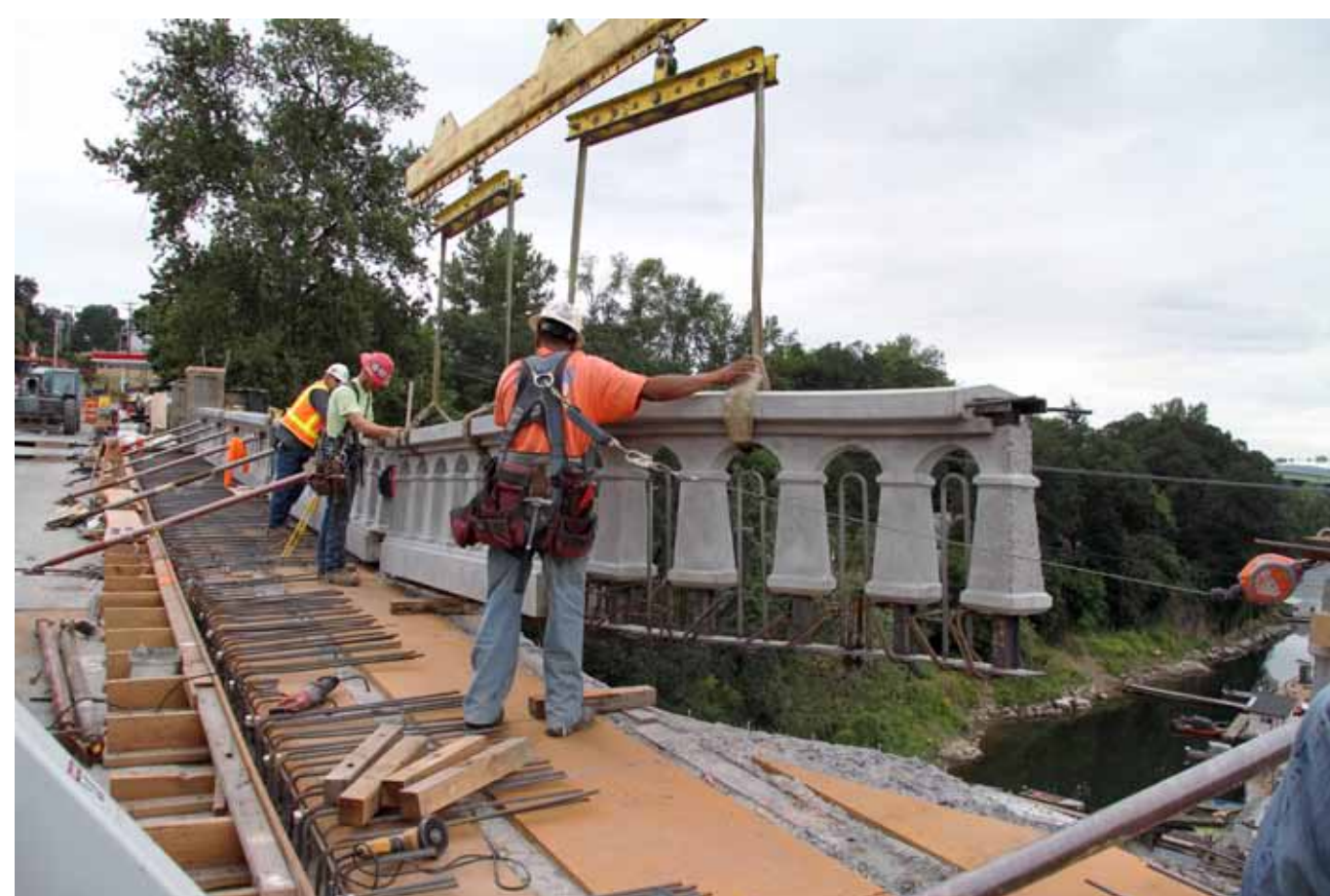
Installing the new railing
