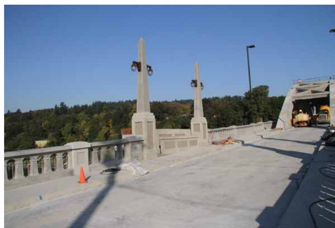
The bridge was last painted in 1983. To create a uniform color ODOT repainted the bridge, choosing a color that closely matched the concrete and the original 1922 color.
