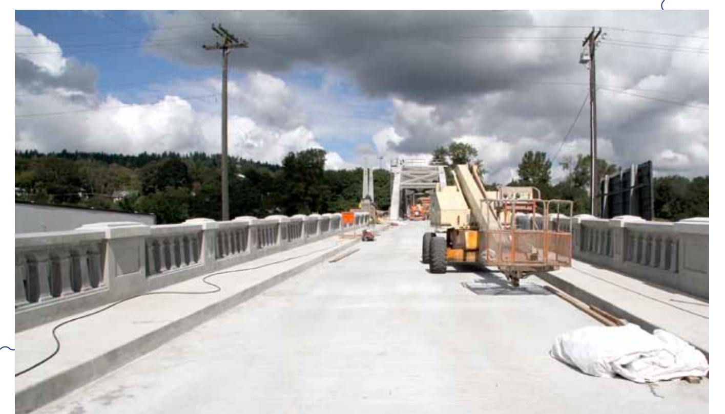
The final railing
