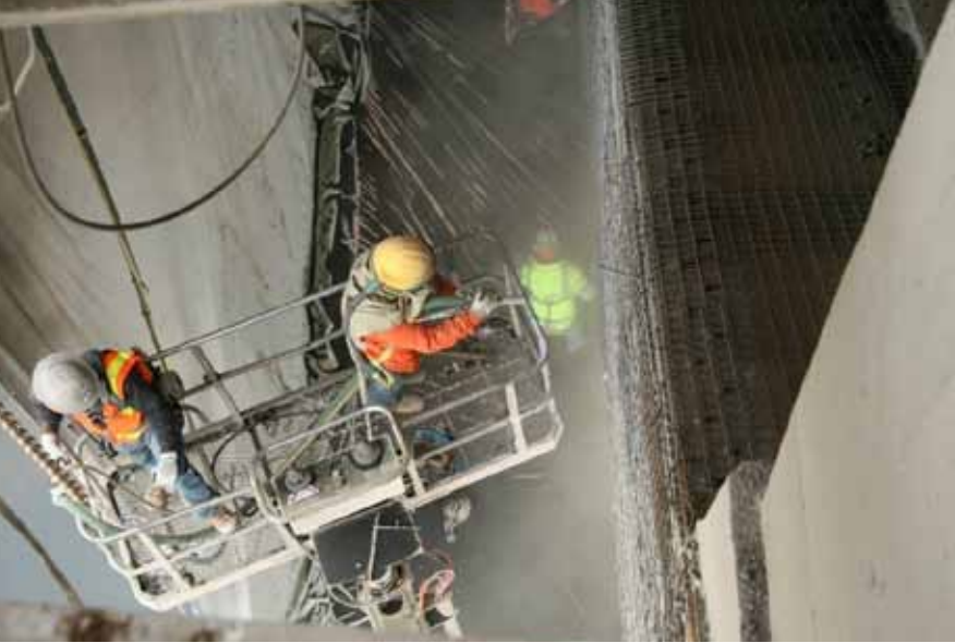
▲ Sandblasting the steel to achieve required surface finish
