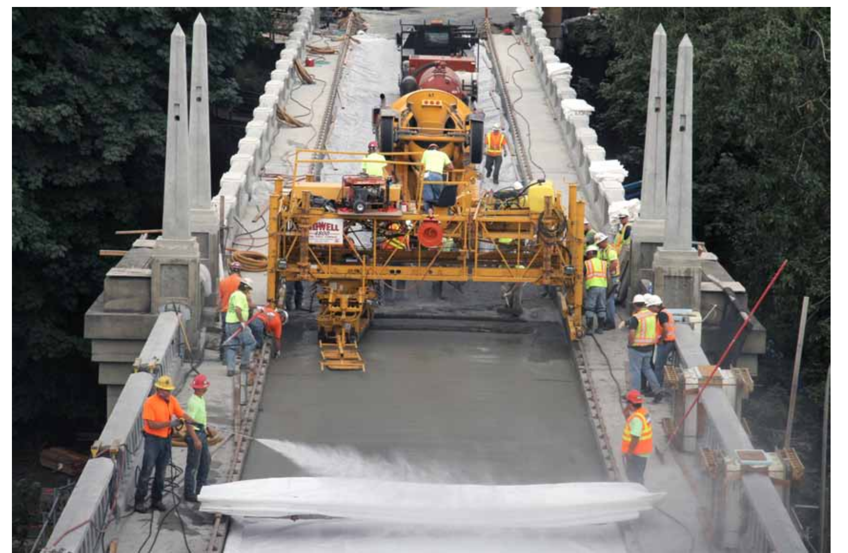
Casting the concrete roadway overlay
