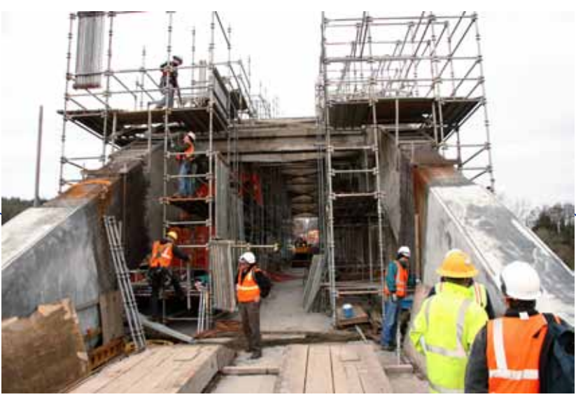
The final shotcrete coating
