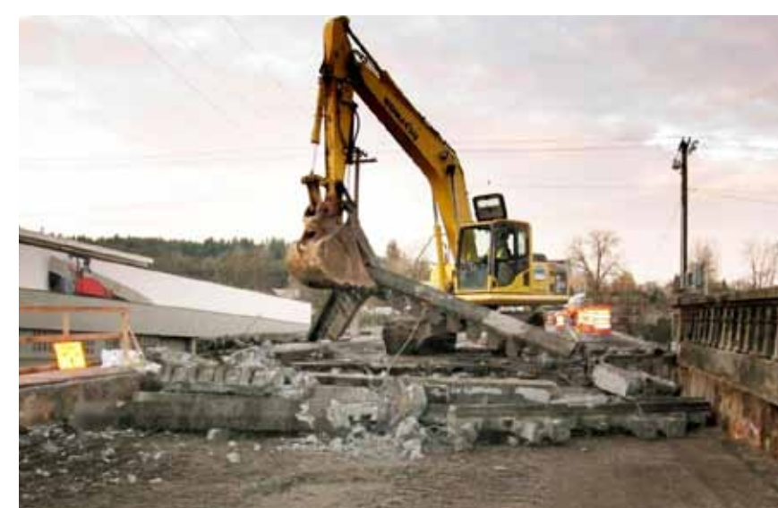
Sidewalks and rails were first removed
