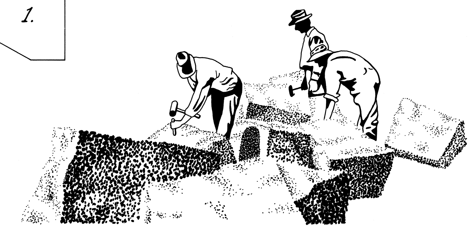
Stone voussoirs were hand cut using templates. Granite was quarried from within the park.
