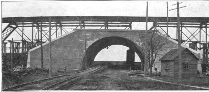
FIG. 5—VIEW SHOWING CYLINDRICAL PIER AND BRIDGE TRUSS MEMBERS UNDER AND EXTENDING THROUGH 60-FT. CONCRETE ARCH.
