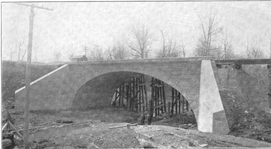
FIG. 7—CONCRETE ARCH BRIDGE OF 75 FT. SPAN, NEAR BRIGHTON, TENN.
