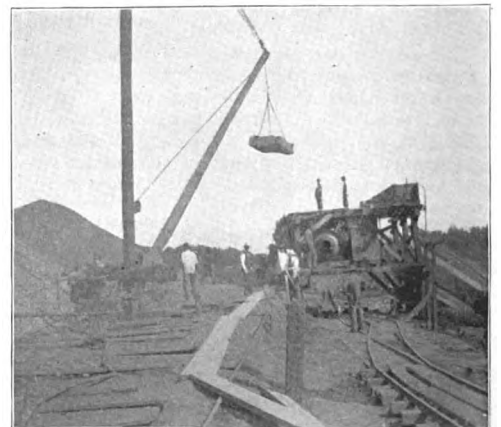
FIG. 8—CONCRETE MIXING PLANT FOR 60-FT. ARCH BRIDGE NEAR BRIGHTON.
