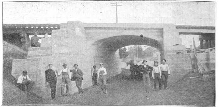
FIG. 13—20-FT. SEGMENTAL CONCRETE ARCH CULVERT.
