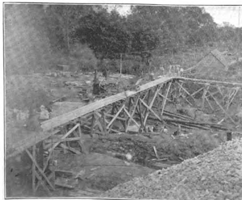
FIG. 9—TRETTLE FOR RUNNING CONCRETE TO PLACE.
