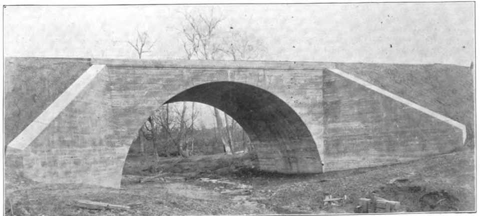
FIG. 11—60 FT. CONCRETE ARCH BRIDGE NEAR BRIGHTON, COMPLETED STRUCTURE.
