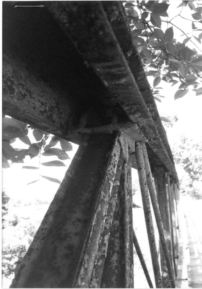
S TRUSS, 2 ND INTERMEDIATE UPPER CHORD PANEL POINT, FROM E
