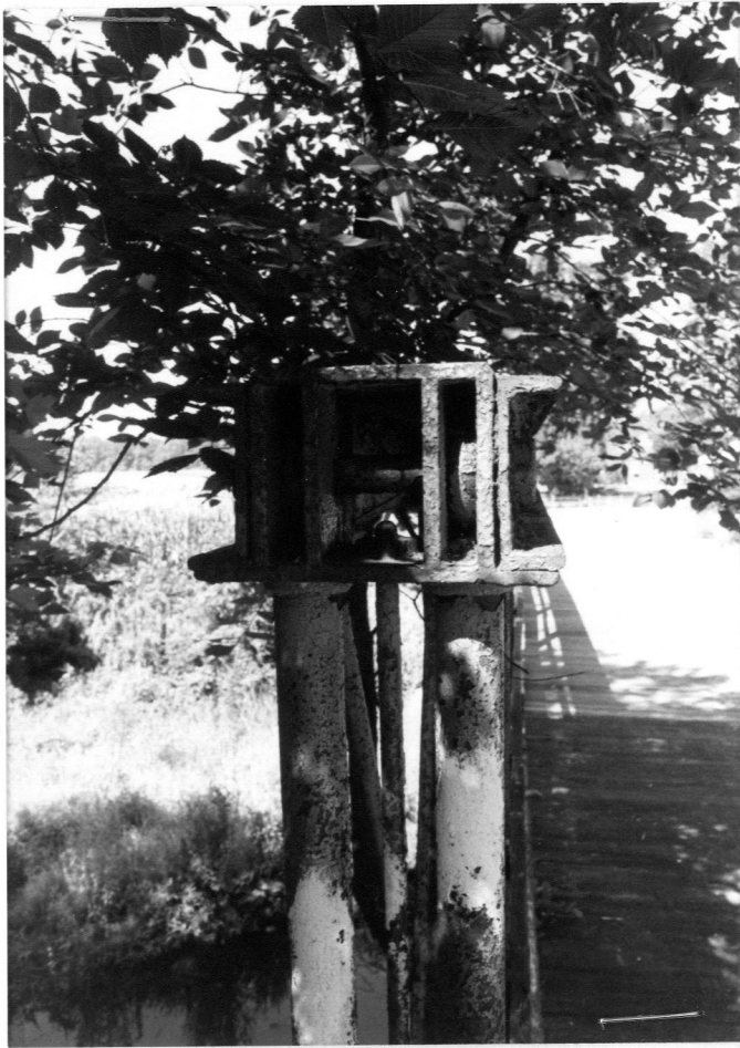
S TRUSS, E ENDPOST UPPER CHORD CONNECTION, FROM E
