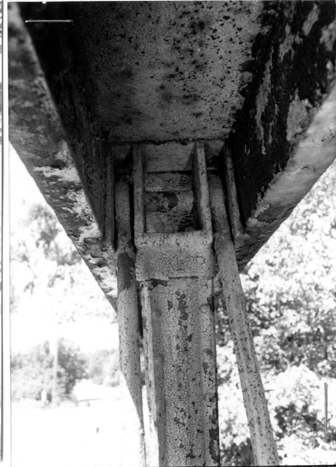
UPPER CHORD INTERMEDIATE PANEL POINT
