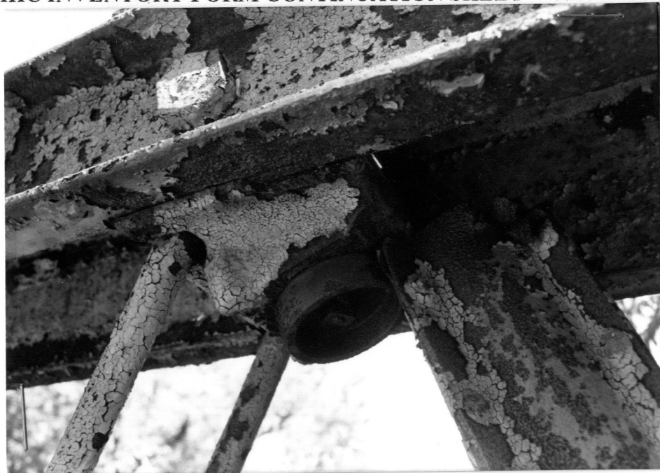
N TRUSS, INTERMEDIATE UPPER CHORD PANEL POINT, WITH DISPLACED POST
