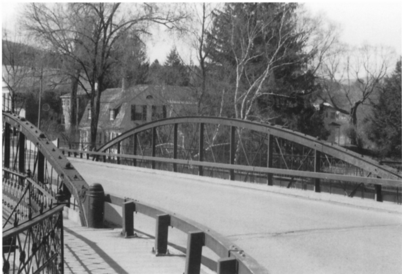
Figure 14. The trusses of the Elm Street Bridge, Woodstock, Vermont, as they are today—preserved as decorative features on the bridge that replaced them. Photo by author, 1995.
