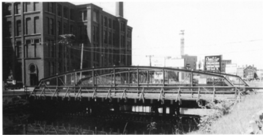
Figure 16. The bridge at Lawrence, Massachusetts, supported by timbers. Photo by author, 1997.
