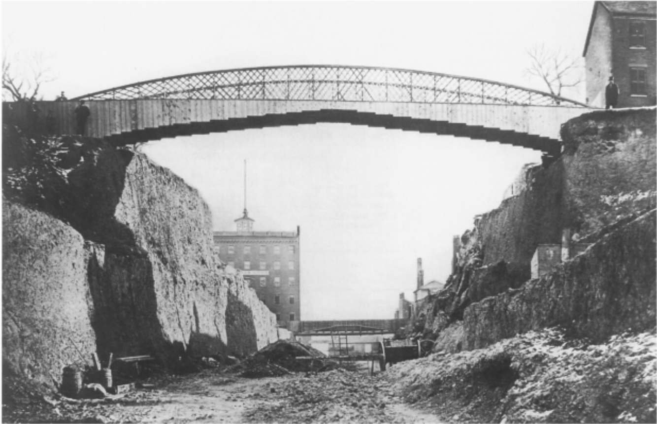
Figure 5. The first bridge built 1868 by the Solid Lever Bridge Company. It carried High Street over Oliver Street as Fort Hill was being cut down. Courtesy of the Bostonian Society/Old State House neg. 1434.
