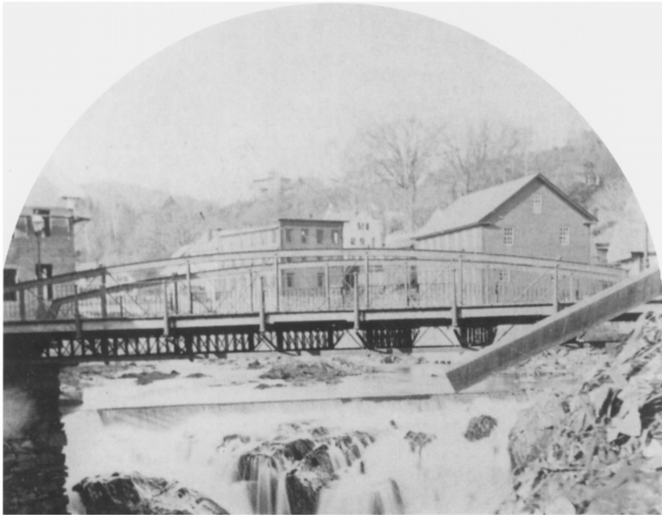
Figure 21. The bridge formerly at Springfield, Vermont. A rare view that shows the transverse trusses that carried the floor in wider trusses. These rested on the bottom chords next to the web posts and cantilever to carry sidewalks outside the roadway. From a stereograph in the collection of Robert M. Vogel.
