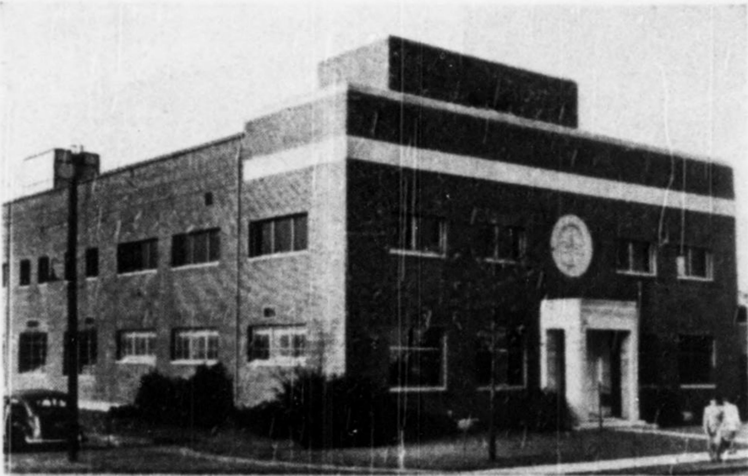
For Merck & Company, M-C & S built a streptomycin plant at Elkton, Va., and simultaneously constructed this processing and packaging plant at Rahway, N. J.
