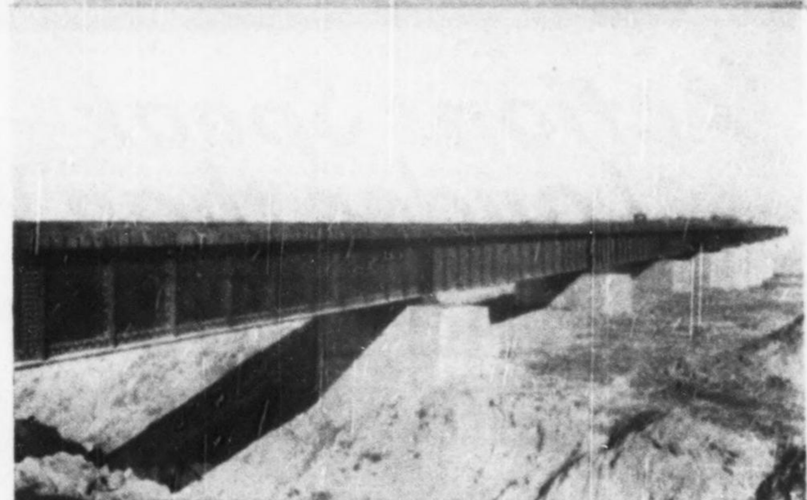
For the Union Pacific Railroad, Merritt-Chapman & Scott constructed 6 grade separation structures and this 11-span bridge at Long Beach, Calif.
