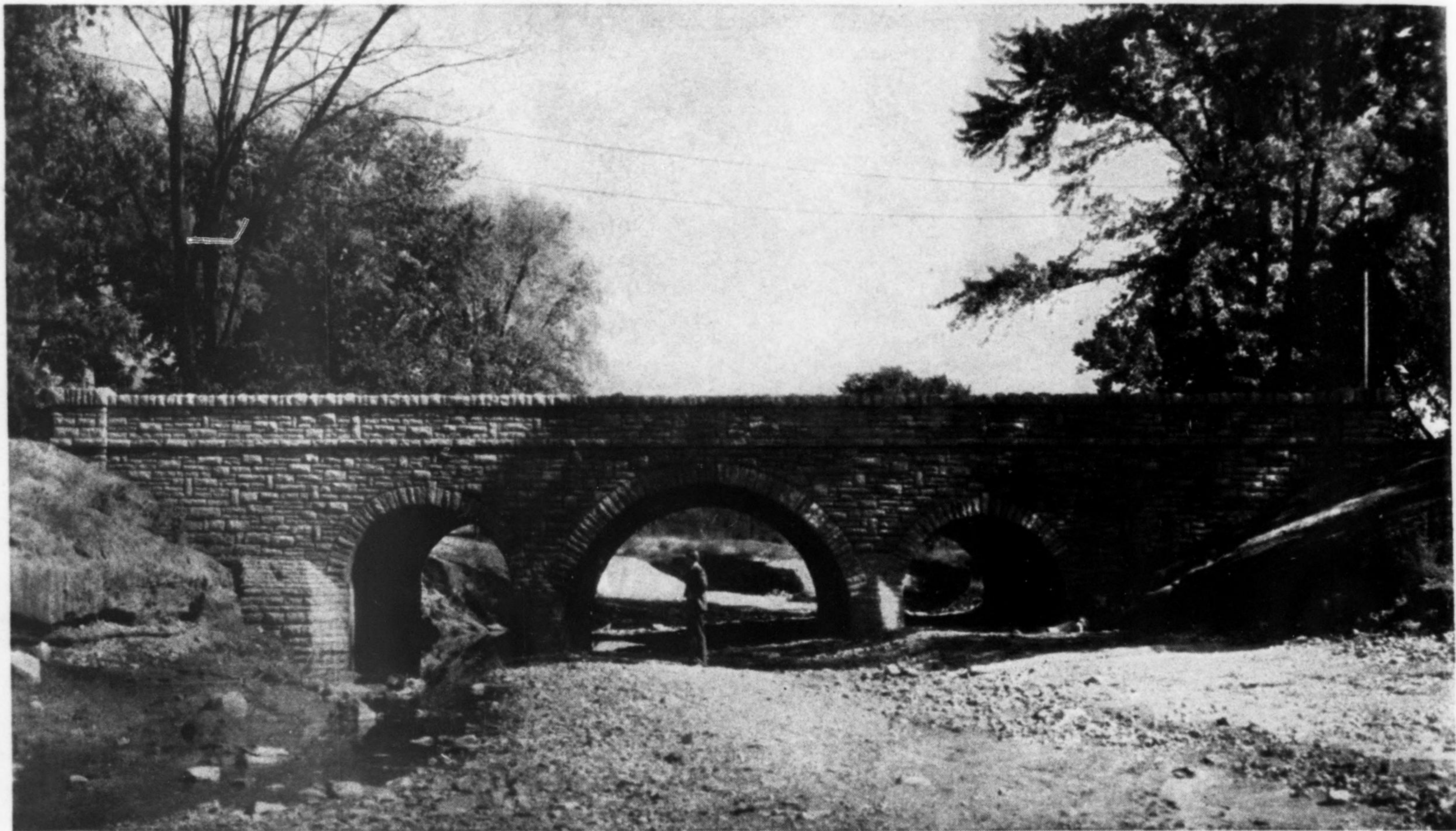
Artistic treatment of stone headwalls on triple Armco MULTI PLATE Arch at Xenia, Ohio.
