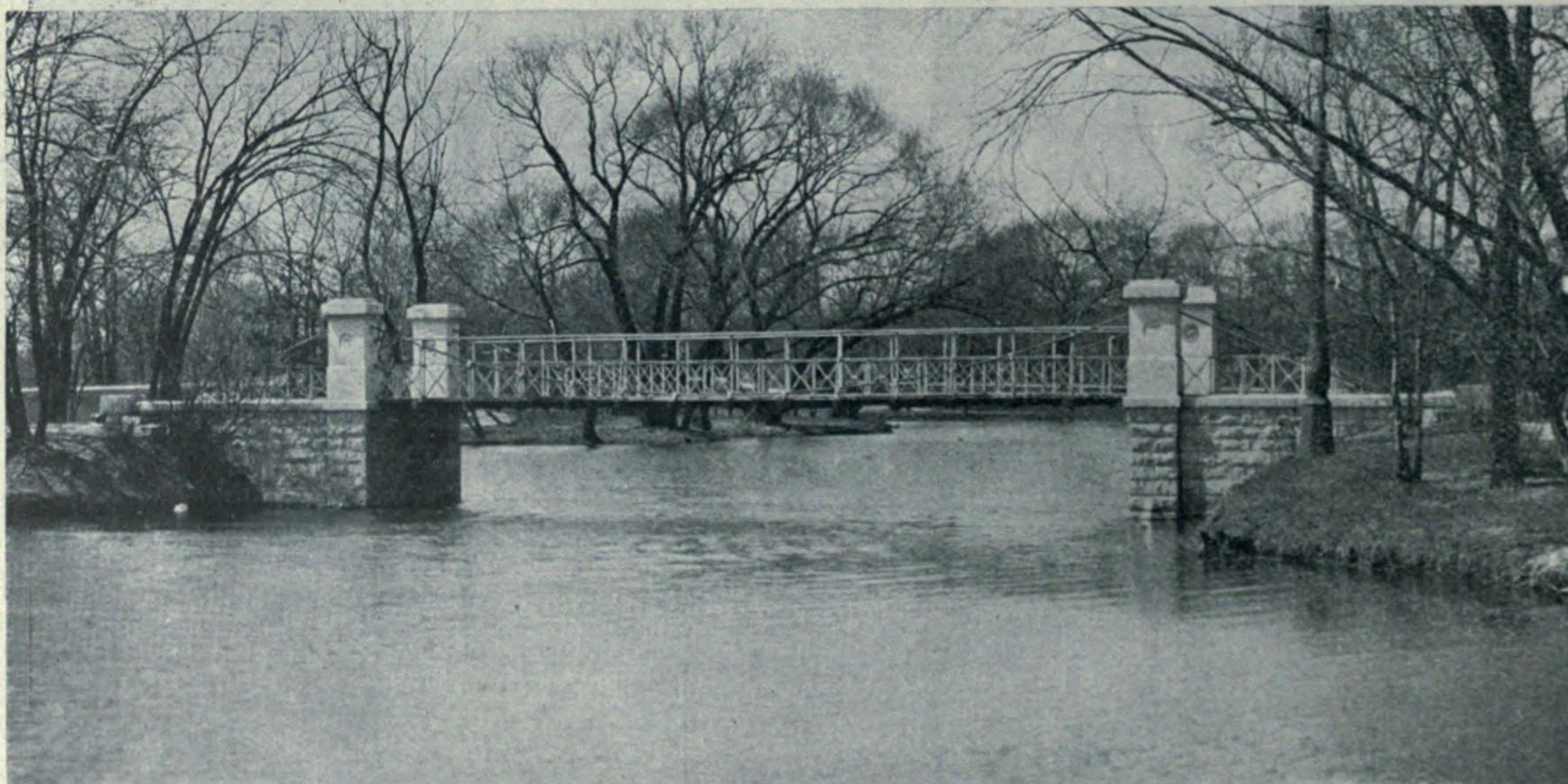
Foot bridge, Garfield Park, Chicago.
