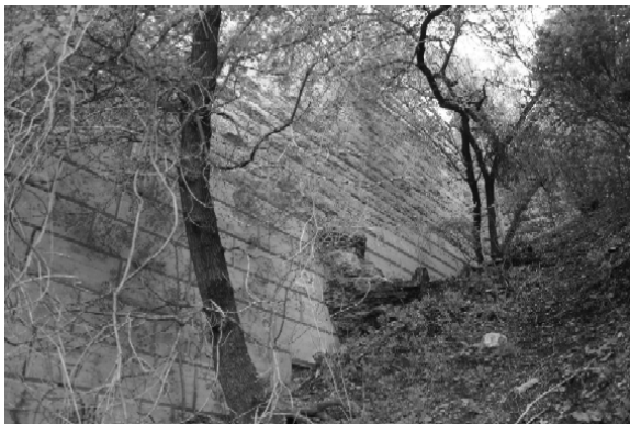
Figure 4. A large portion of the south face of the east abutment has been repaired with concrete.
