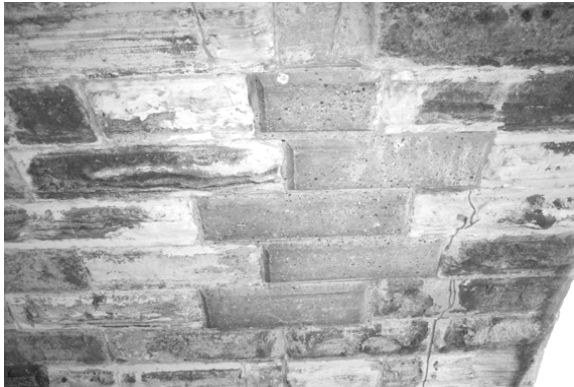
Figure 2. Typical concrete repairs to stone masonry of intrados. The repairs do not appear to be new or recent. The concrete is carefully formed to represent the shape of the stone block that it replaces.
