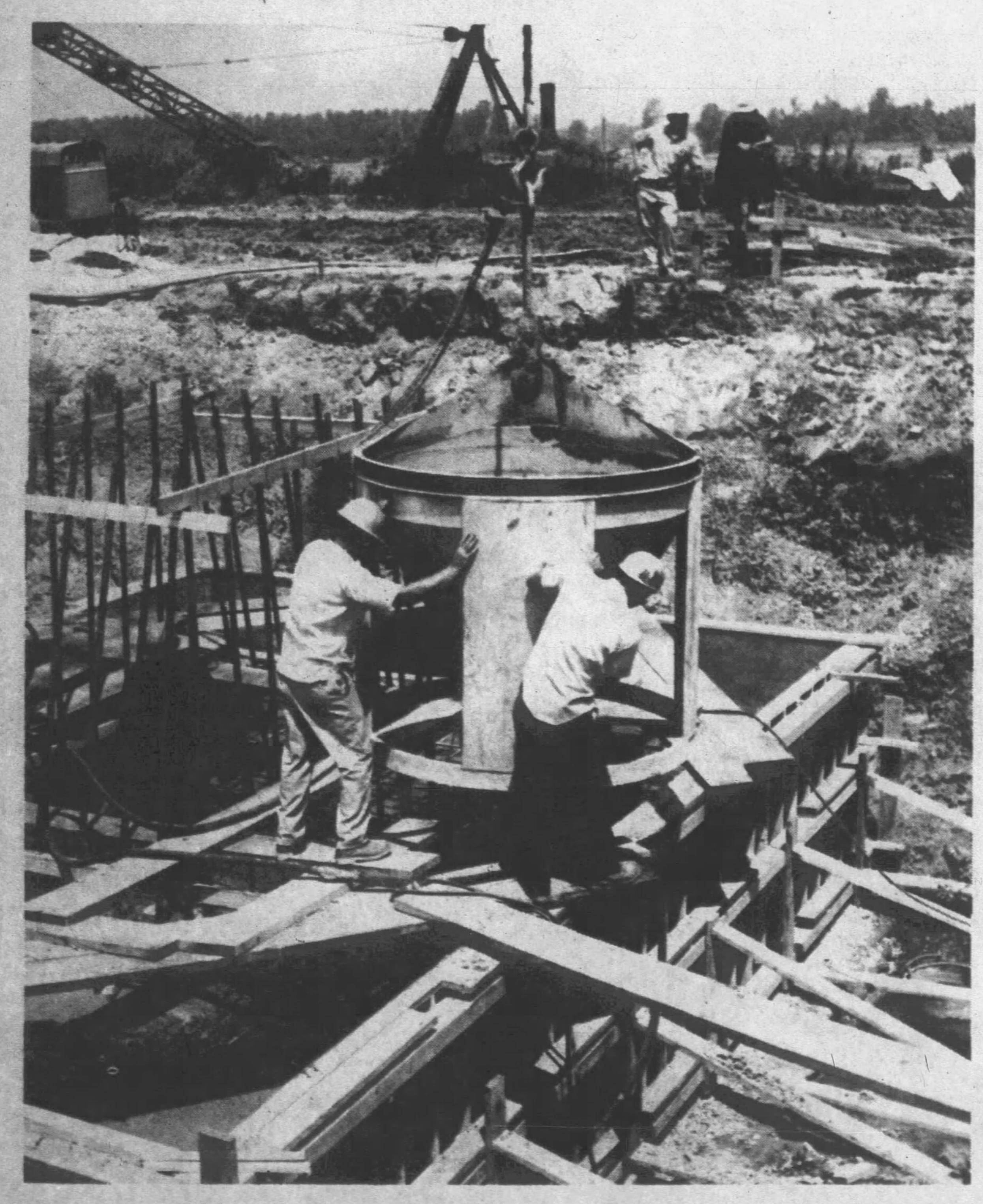
WORKMEN ARE NOW pouring concrete on the new 7,098-foot Mississippi River bridge near Caruthersville. Work on this first phase of the construction is about 20 per cent complete. The bridge on Interstate Route 155 is being built in cooperation with Tennessee.
