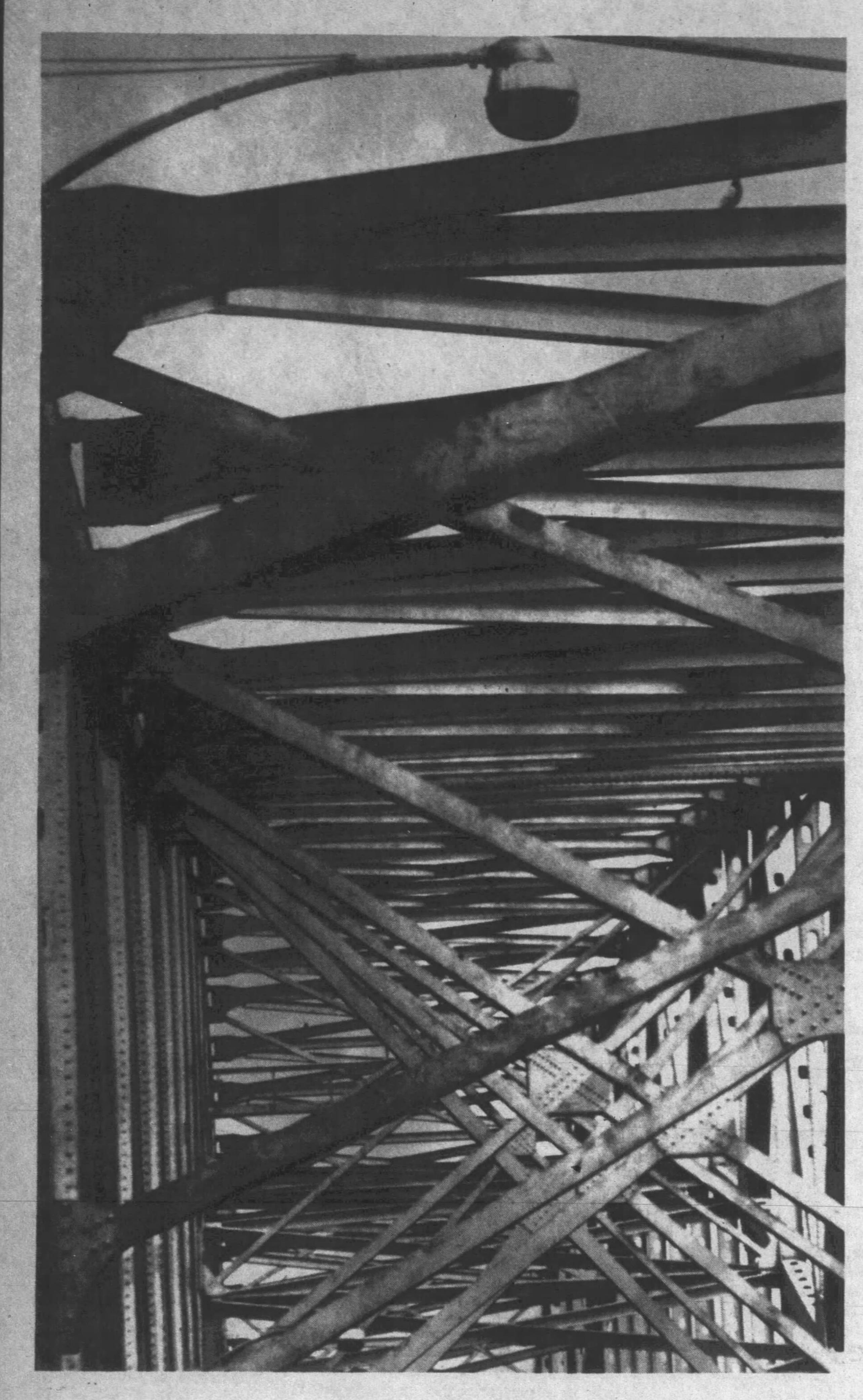
TO A NONOBSERVANT MOTORIST, the network of girders in a bridge's superstructure IS the bridge. Actually, it's one of the simpler problems of bridge building. Most of the engineering and design problems, as well as cost and labor, are found below.
