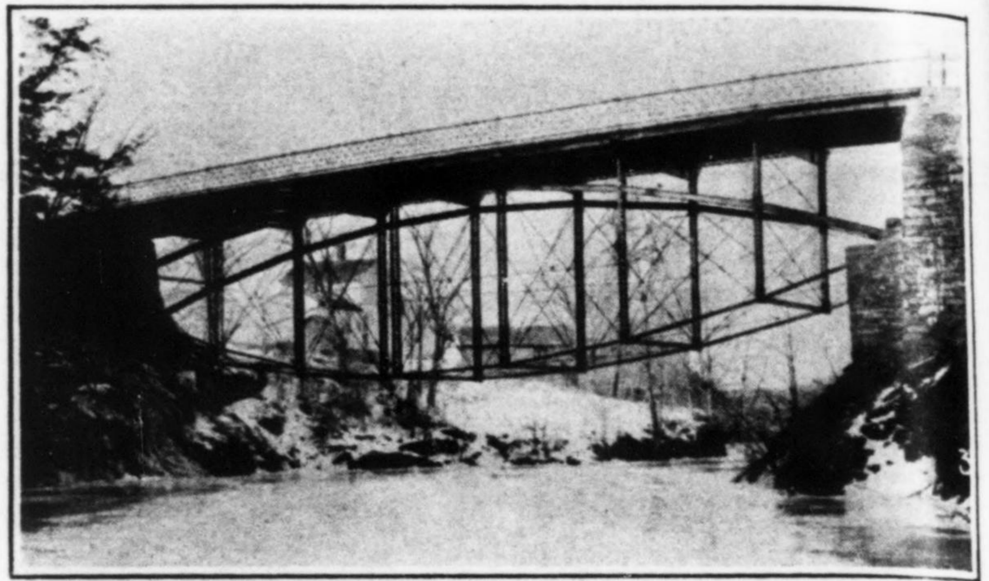
FIG. 3—DECK PARABOLIC TRUSS AT SUFFIELD, CONN.
