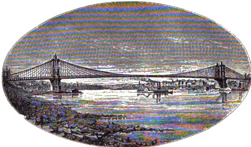
Collington and Cincinnati Suspension Bridge, built by JOHN A. ROEBLING. Main Span, 1,067 feet.
