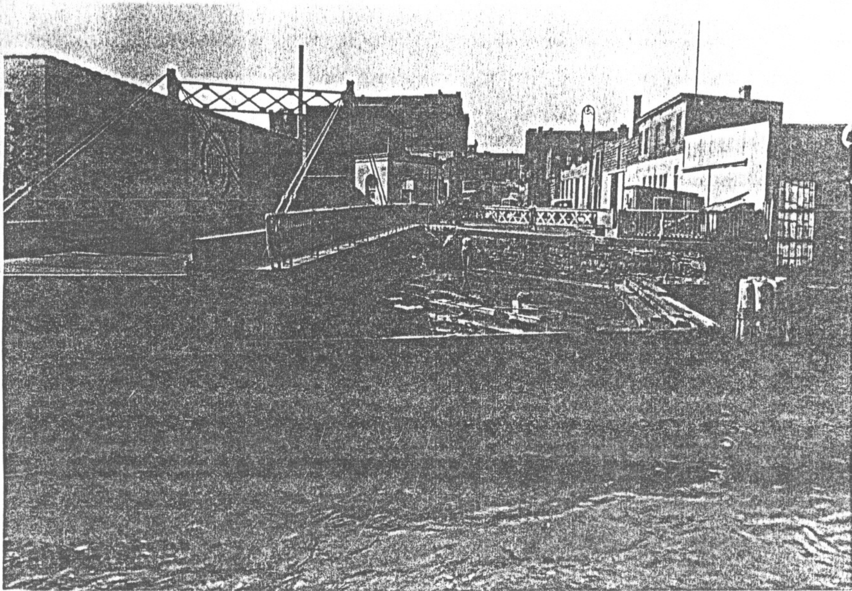
CARROLL STREET BRIDGE, over the Gowanus Canal, Brooklyn Built: 1888-89
