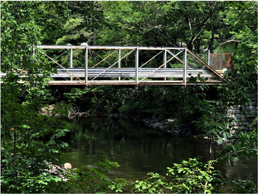
Photo 8. Old Schroon River Bridge to be replaced, Structure 3. View southwest.
