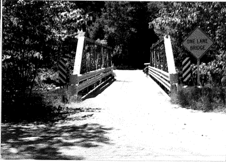
End roadway approach looking west on connecting road.
