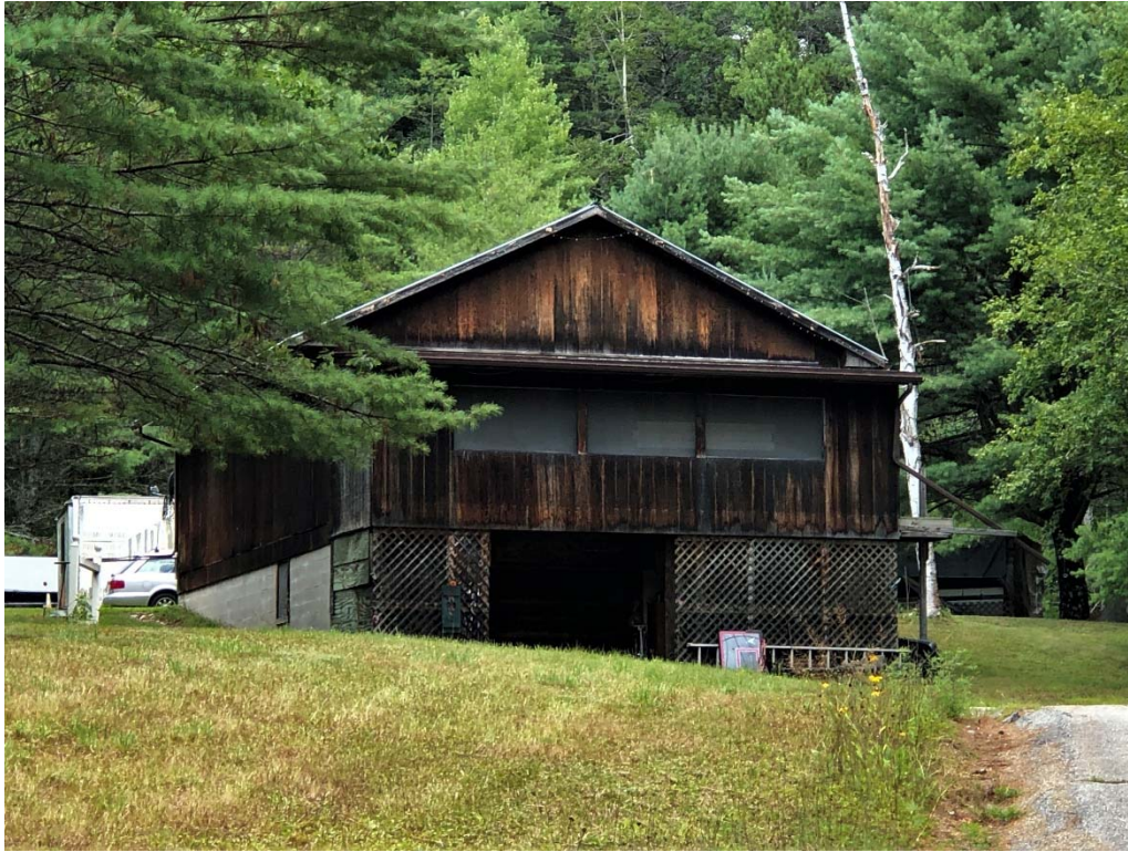
Photo 3. 2549 Schroon River Road garage, Structure 1b. View west.
