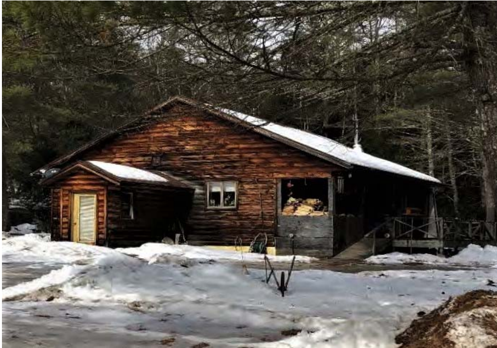
Photo 1. 2549 Schroon River Road, Structure 1a. View northwest.
