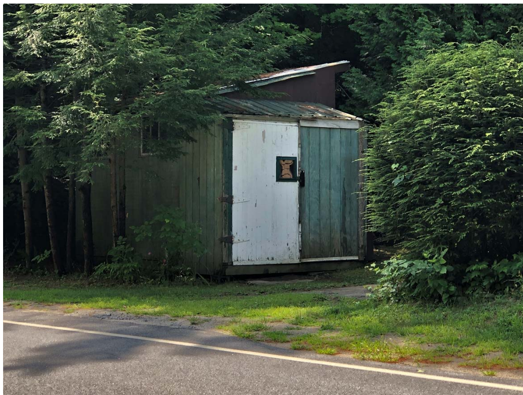
Photo 16. 2057 Schroon River Road garage, Structure 6b. View south.
