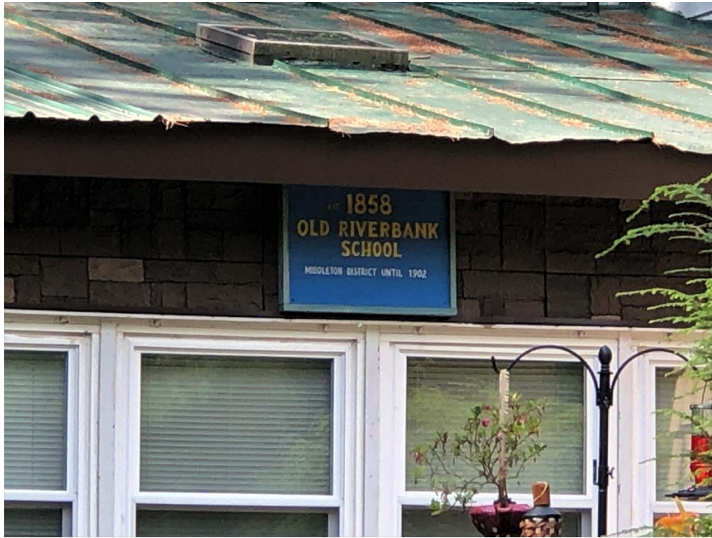
Photo 15. Sign on 2057 Schroon River Road, Structure 6a. View west.
