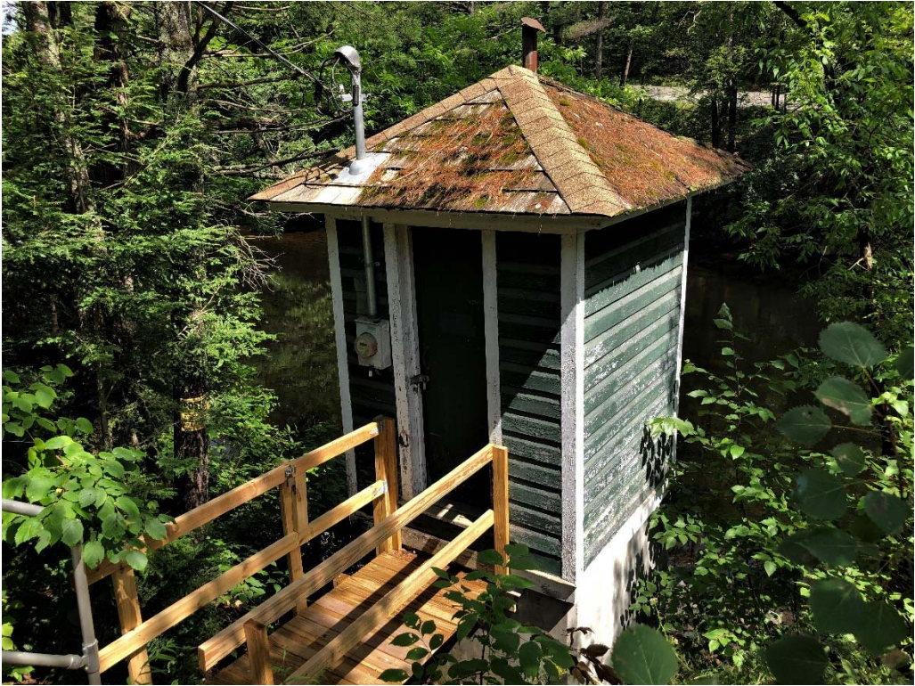
Photo 11. USGS gage house, Structure 4. View southwest.
