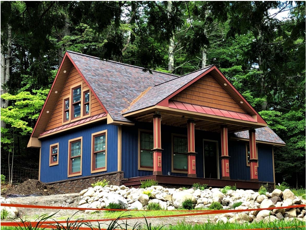
Photo 12. 2039 Schroon River Road, Structure 5. View west.
