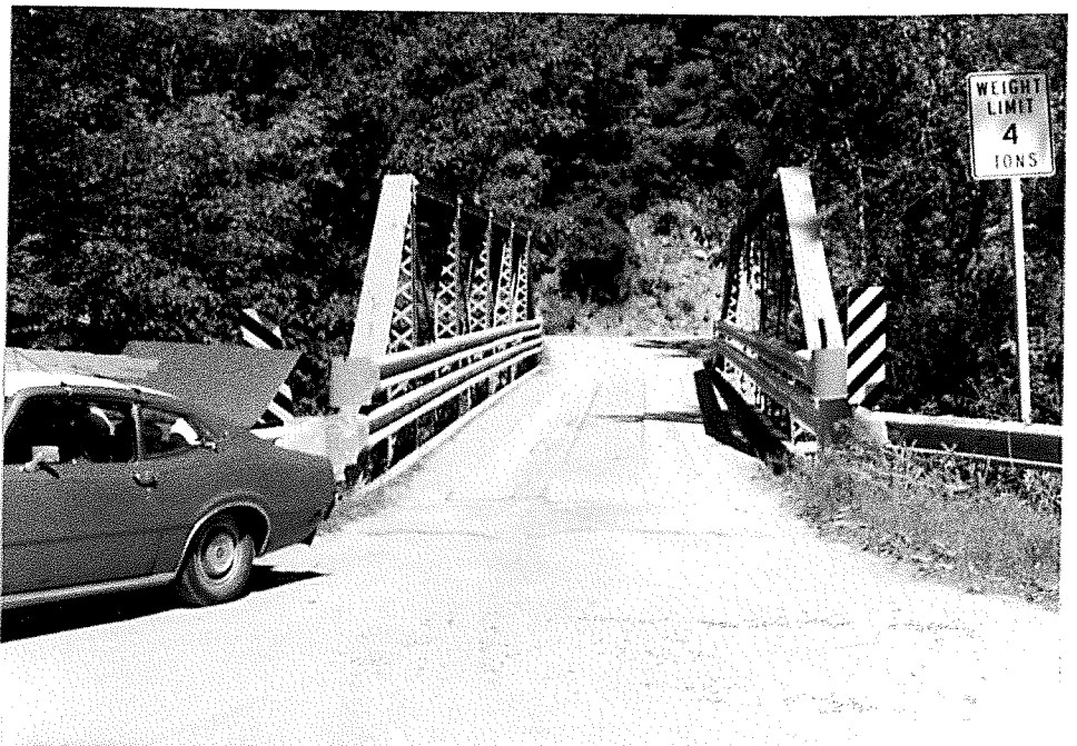
Beginning roadway approach looking east on connecting road.
