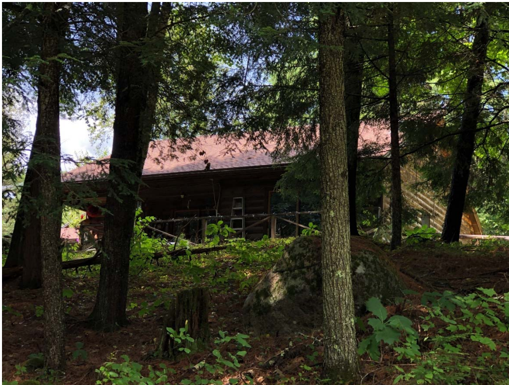
Photo 2. 2549 Schroon River Road, Structure 1a. View west.
