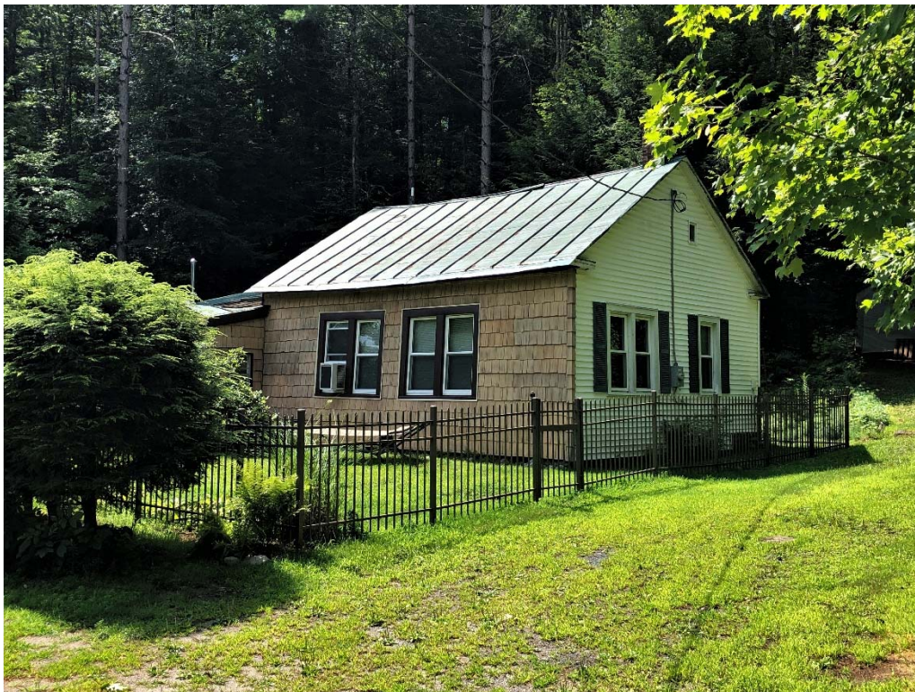
Photo 14. 2057 Schroon River Road, Structure 6a. View south.
