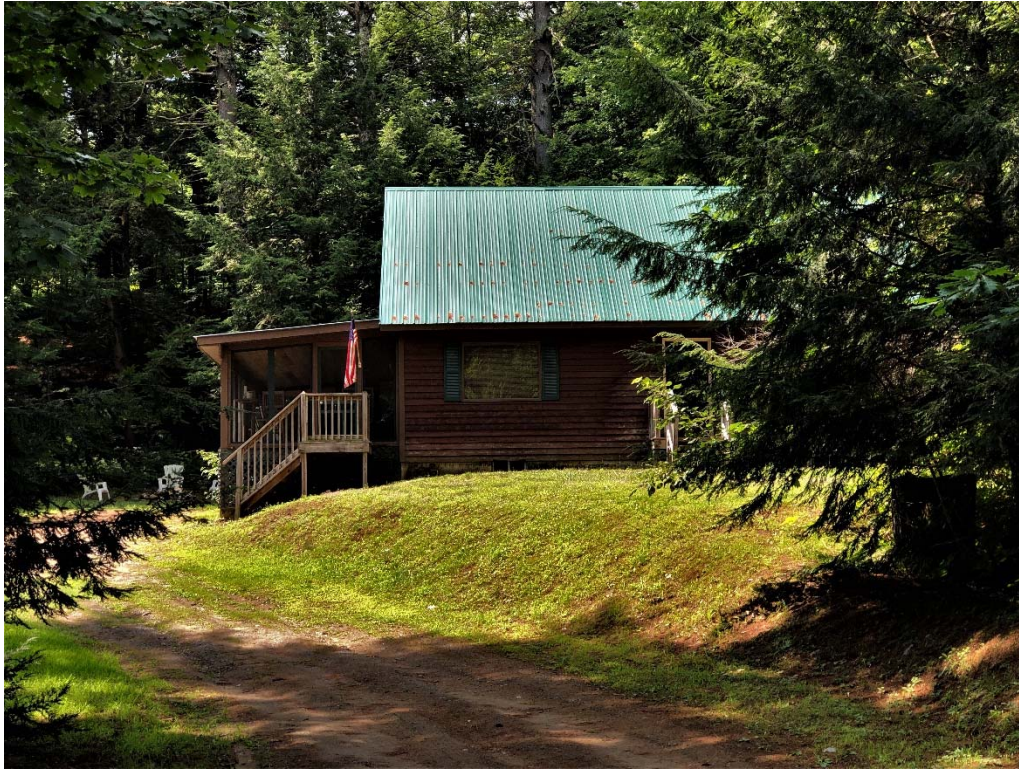
Photo 17. 2067 Schroon River Road, Structure 7. View southwest.
