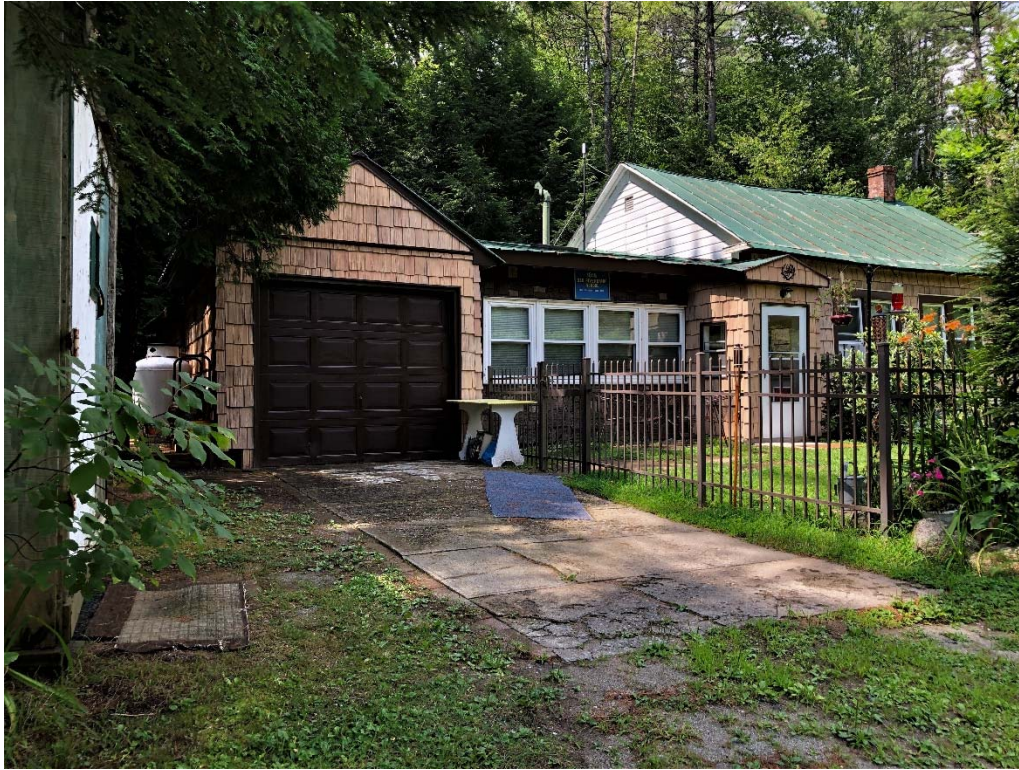
Photo 13. 2057 Schroon River Road, Structure 6a. View west.
