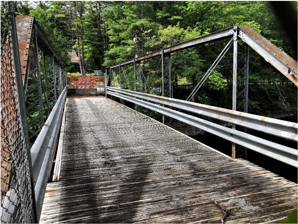
Photo 7. Old Schroon River Bridge to be replaced, Structure 3. View southwest.
