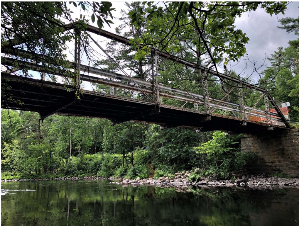
Photo 6. Old Schroon River Bridge to be replaced, Structure 3. View south.
