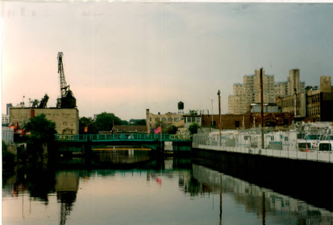
VIEW LOOKING North DESCRIPTION Union Street Bridge over Gowanus Canal- south elevation (BIN # 2-24027-0)
