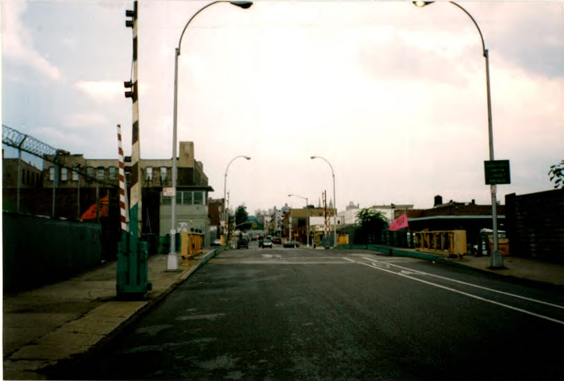
VIEW LOOKING East PHOTO NO. 3 DESCRIPTION Union Street Bridge over Gowanus Canal- top of bridge (BIN # 2-24027-0)
