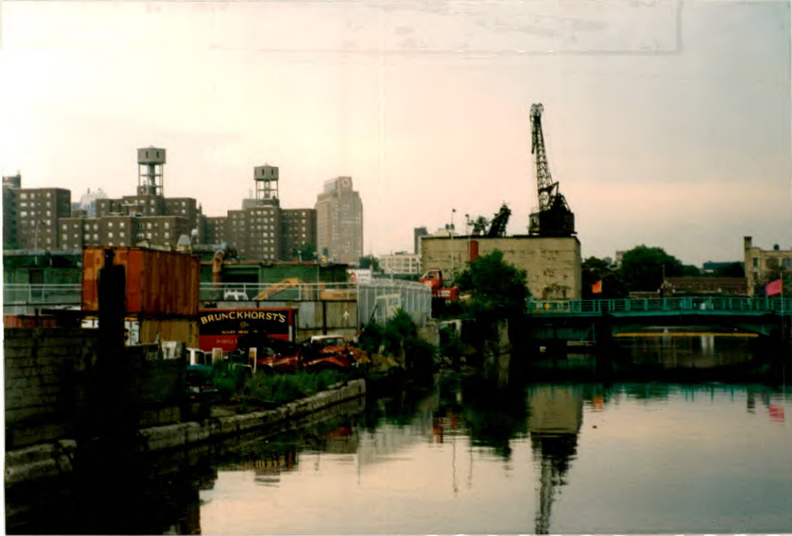
VIEW LOOKING North DESCRIPTION Union Street Bridge over Gowanus Canal- south elevation (BIN # 2-24027-0)
