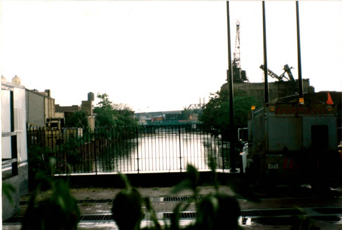
VIEW LOOKING South PHOTO NO. 5 DESCRIPTION Union Street Bridge over Gowanus Canal- north elevation (BIN # 2-24027-0)
