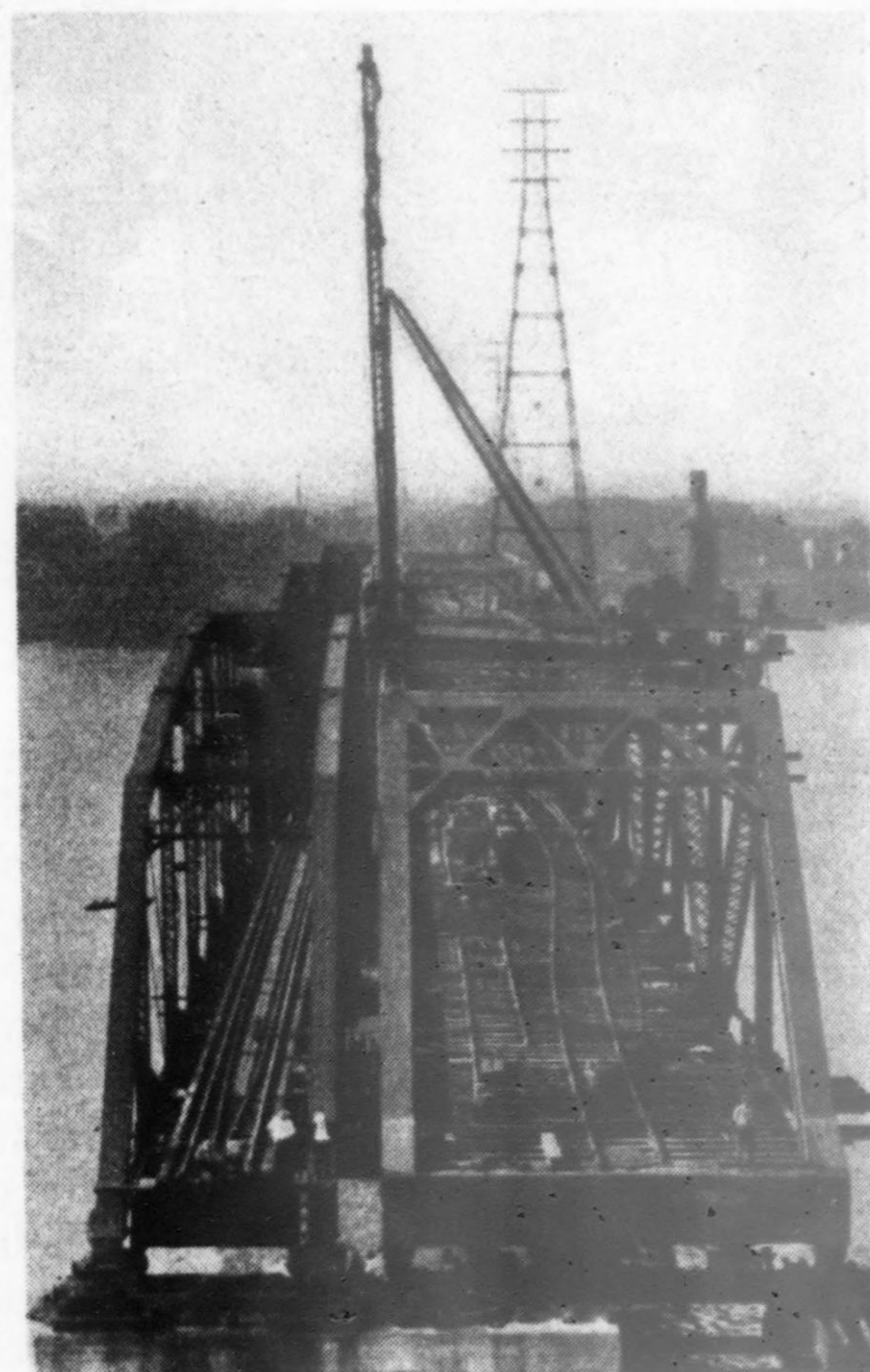
After the New Spans Had Been Erected to the Right of the Old Spans, Cantilever Beams Hung Under the New Spans Were Used to Support the Old Spans During the Lateral Shift and While the Old Spans Were Being Dismantled
