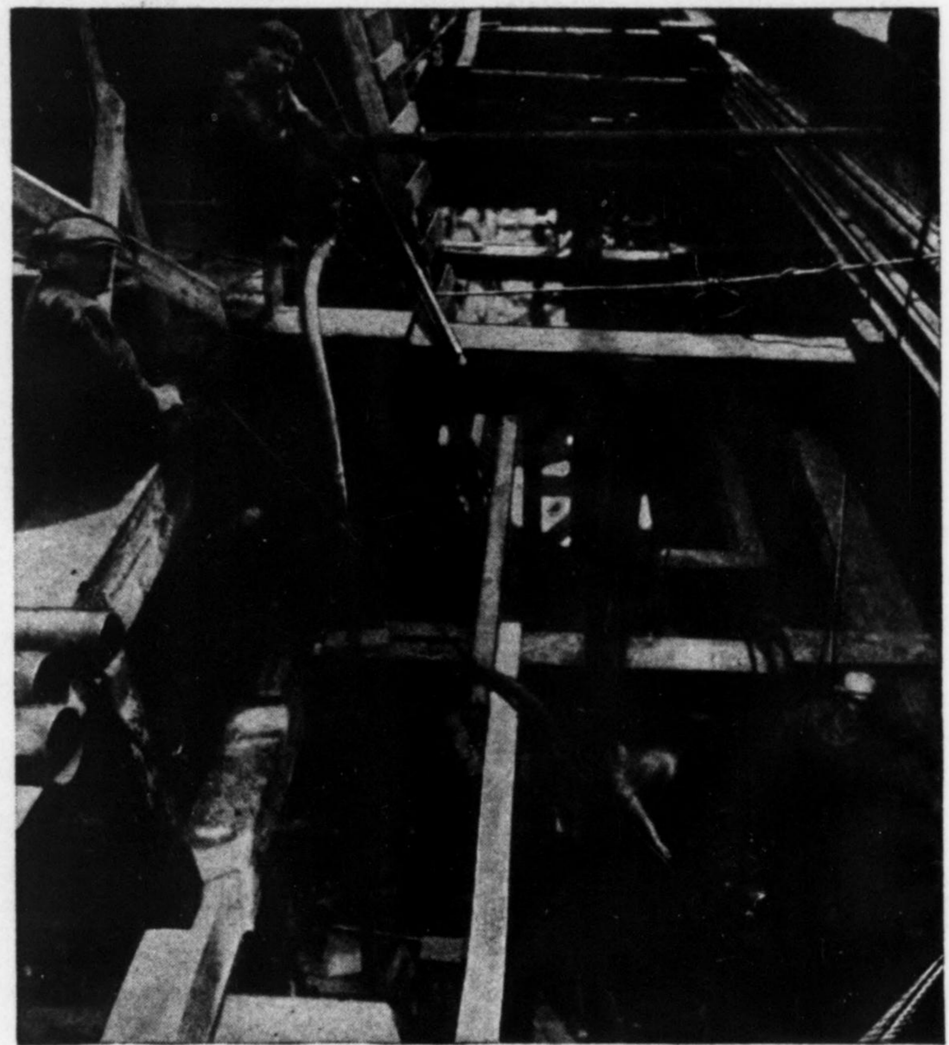
FIG. 2—DEWATERED COFFERDAM INCLOSING OLD PIER
