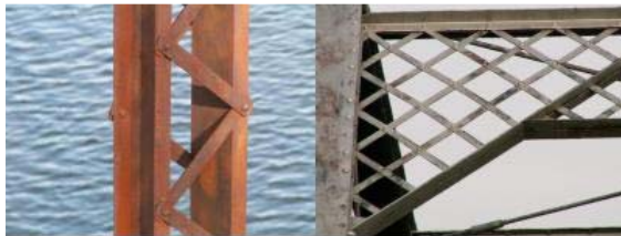
V-lacing on built-up beam | Lattice on portal bracing.
