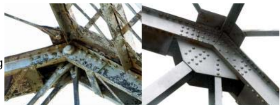
Pinned connection. | Riveted connection.
