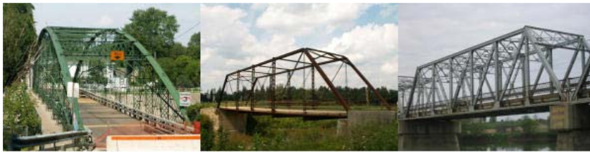
A bowstring truss bridge. | A pin connected truss bridge. | A rivet connected truss bridge.
