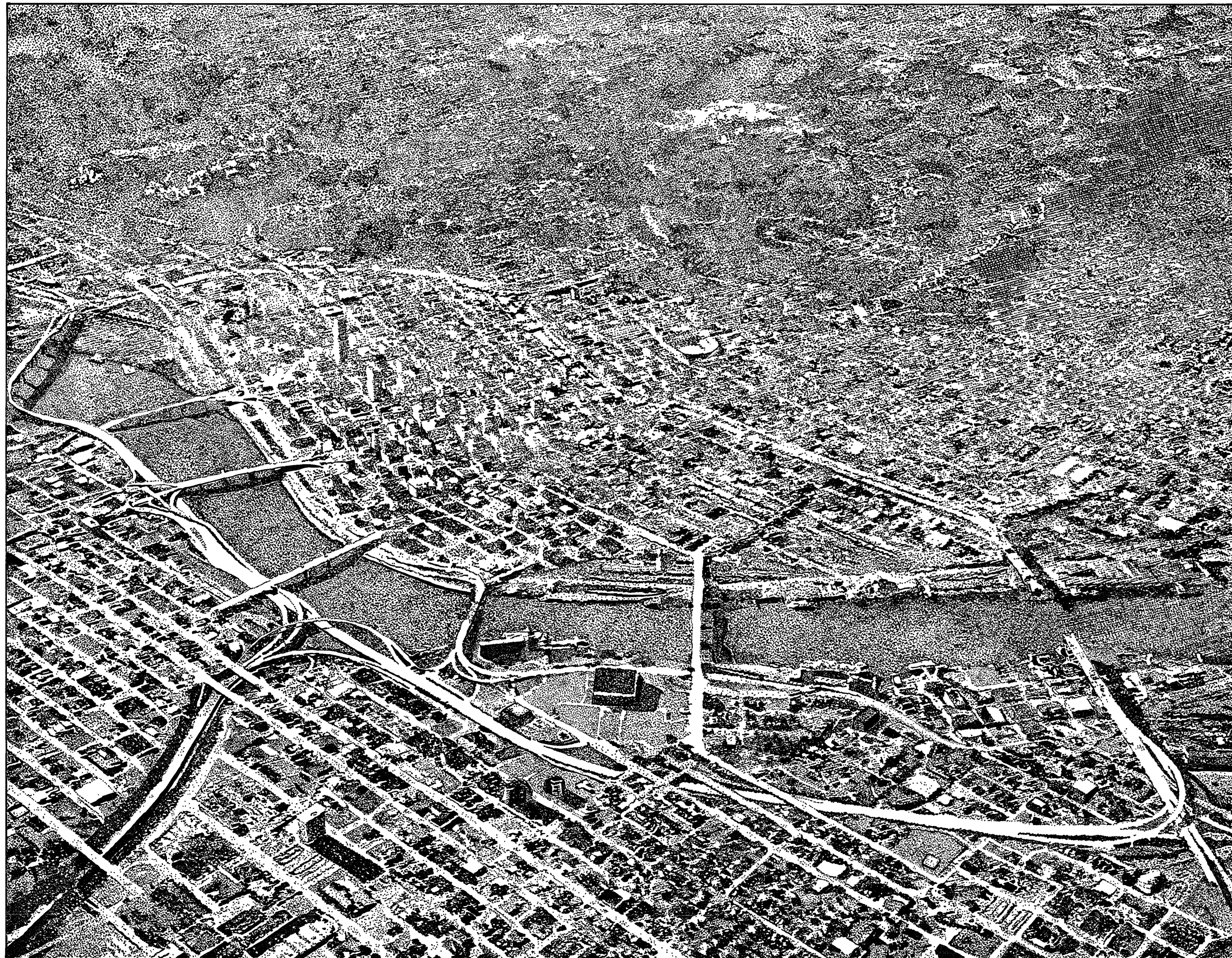
This image shows the city loop formed by the Interstate 5 and 405 freeways. The Fremont Bridge which will complete the loop is under construction (far right.) Courtesy of Oregon Department of Transportation, 1972.
