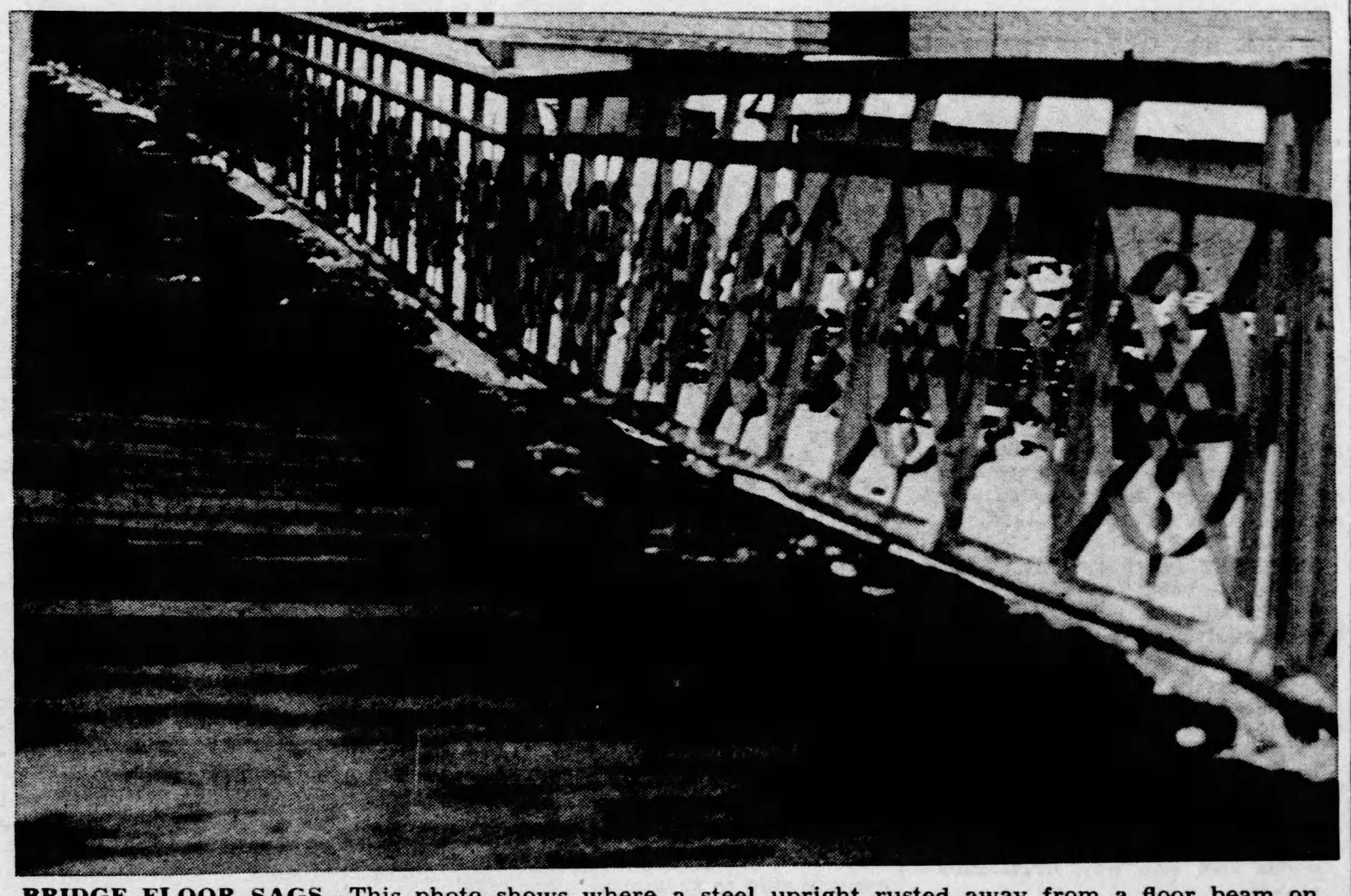
BRIDGE FLOOR SAGS—This photo shows where a steel upright rusted away from a floor beam on the Tenth street bridge this noon, causing the bridge floor on the east side to sag about six inches. If a heavy truck had passed before the break was noticed, it might have caused the entire structure to give way, City Manager Jay F. Gibbs said. The bridge is closed until repairs can be made and the rest of the beams checked. (Times Herald Staff Photo)
