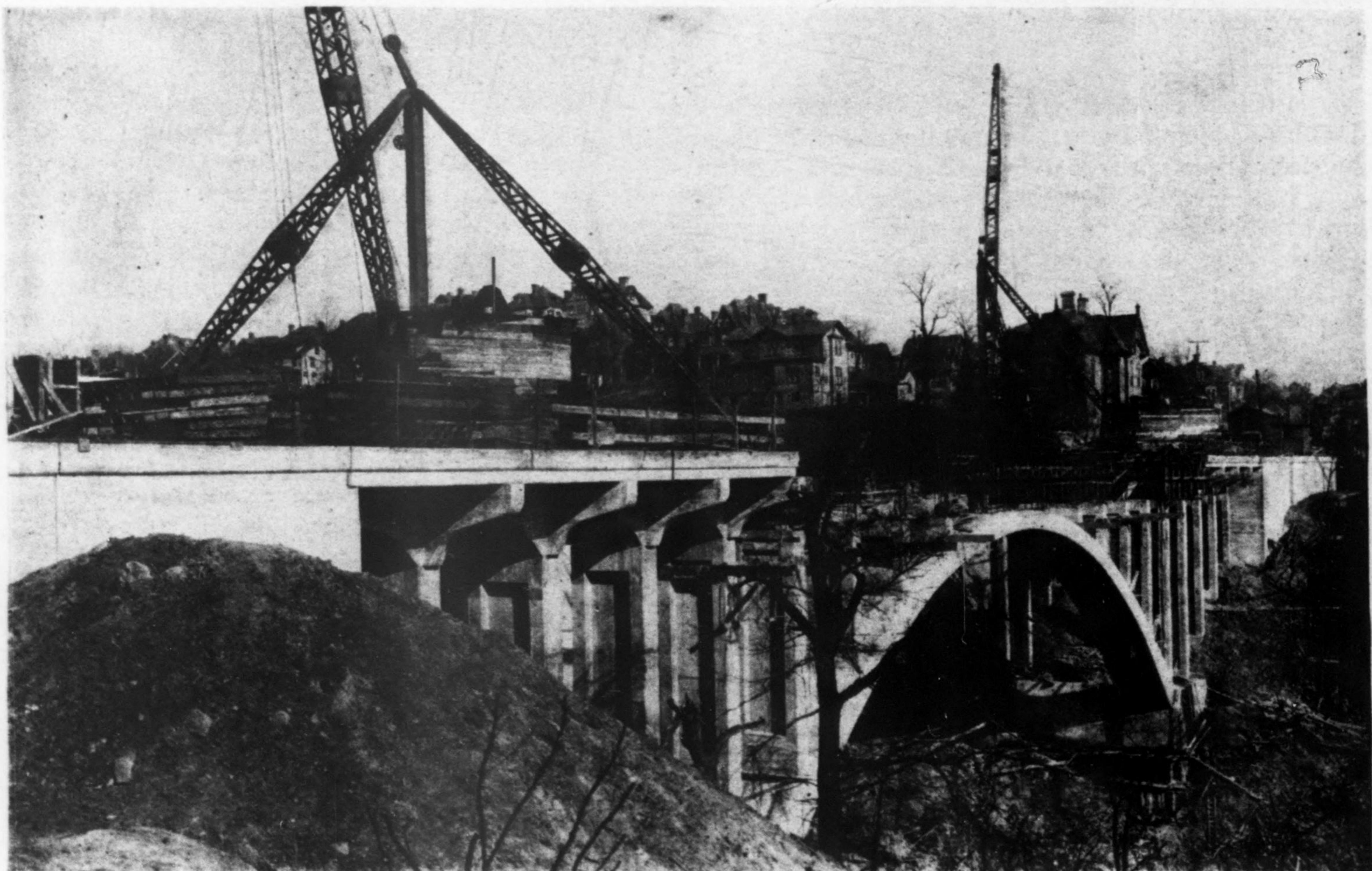
DERRICKS ON APPROACHES, FREMONT ST. ARCH
