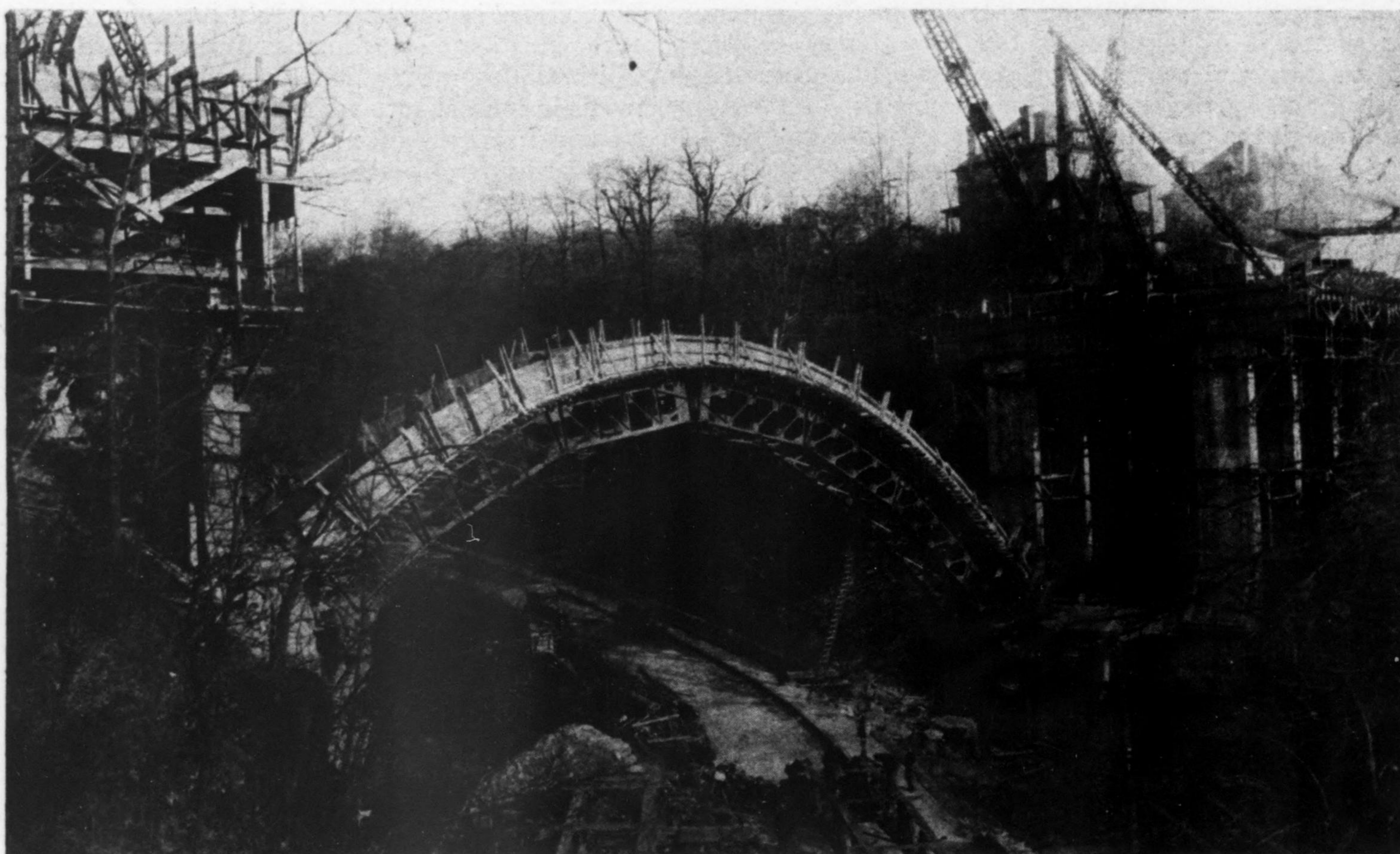
CENTERS AND ARCH-RIB FORMS, DILWORTH RUN BRIDGE
