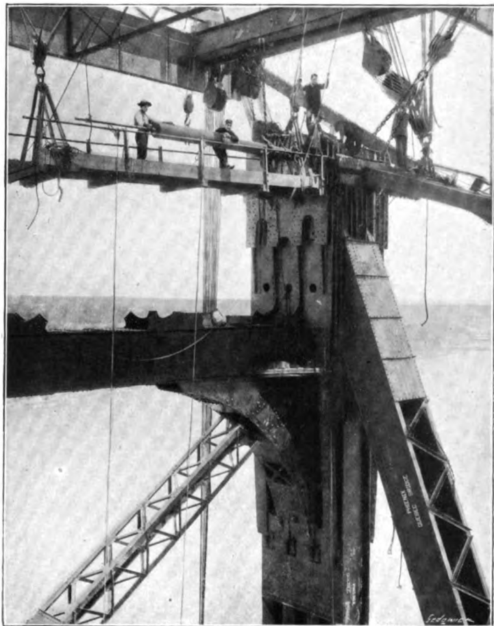
FIG. 11. DRIVING MAIN 12-IN. TOP CENTRE-PIN.
