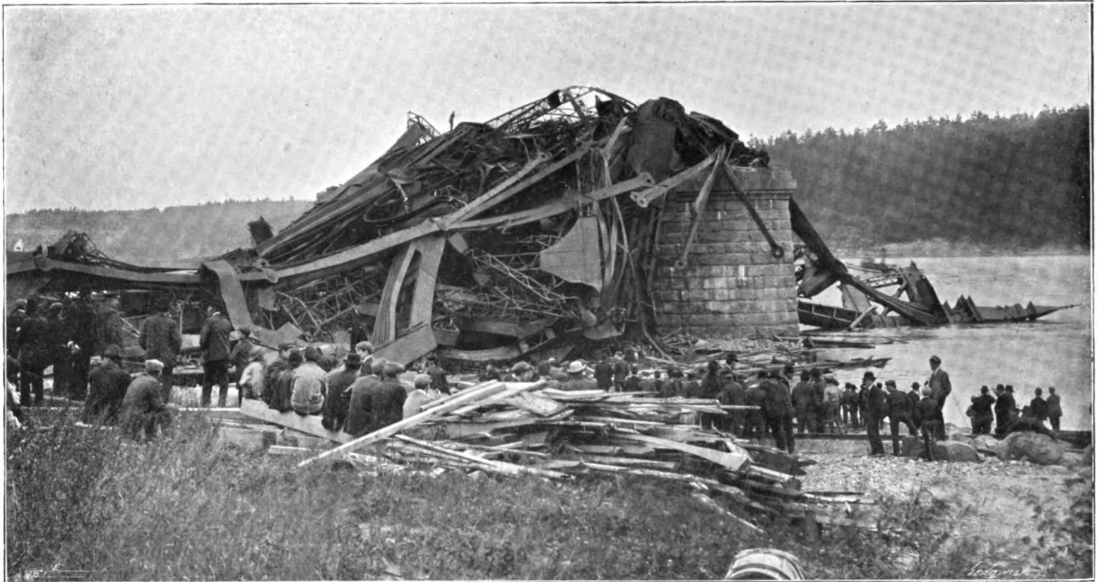
FIG. 3. BROKEN STEEL-WORK PILED OVER AND AROUND THE RIVER PIER.
