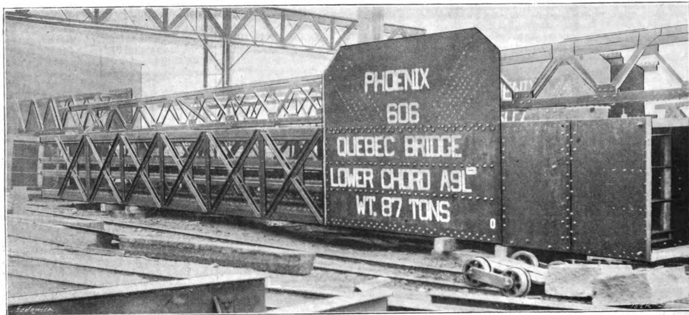
FIG. 71. SECTION 9 OF LEFT-HAND LOWER CHORD OF ANCHOR-ARM.
