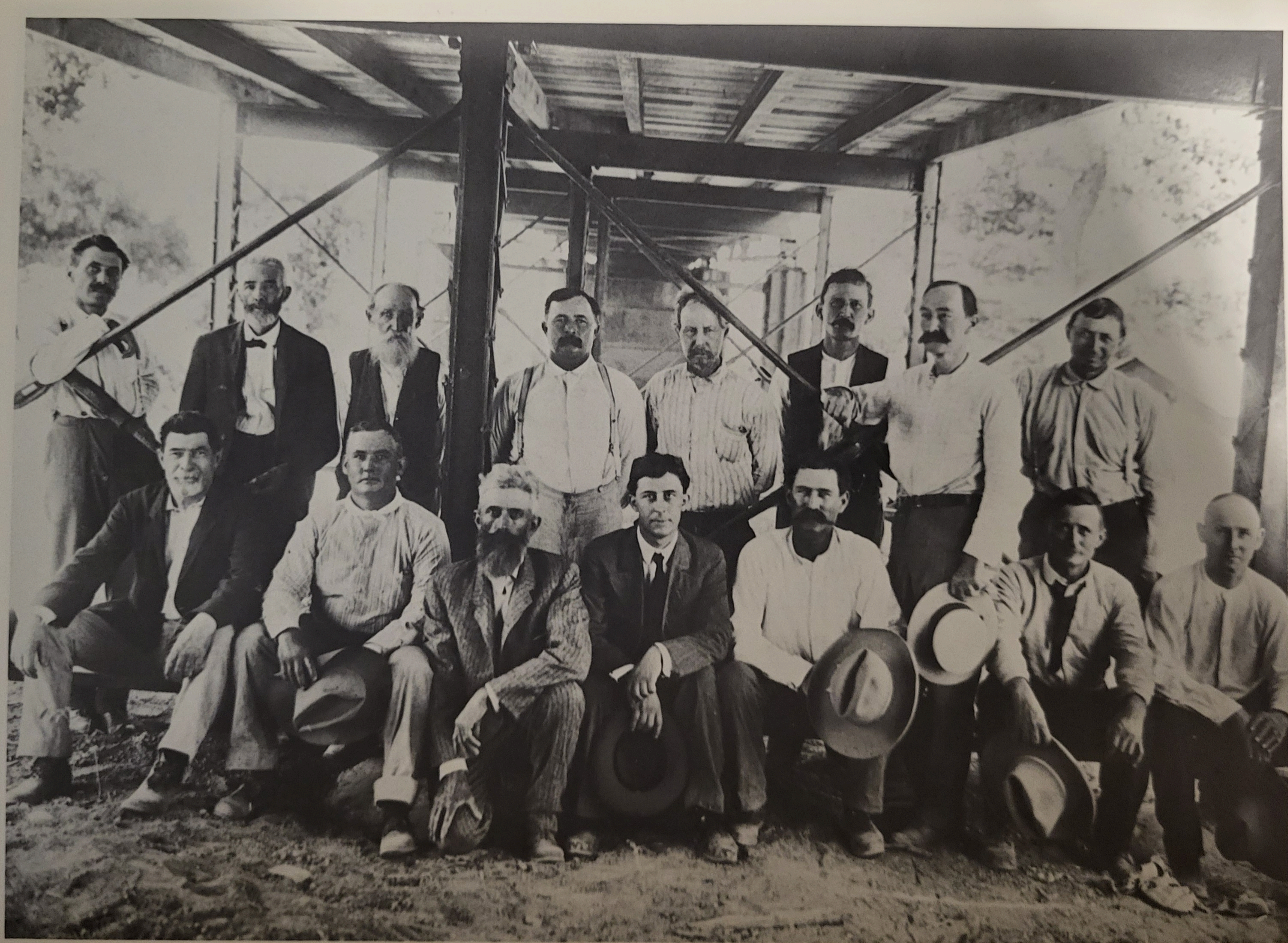
The Guadalupe County Commissioners, engineers, and others responsible for the building of the bridge over the Guadalupe River at McQueeney. Third from right on back row under uncompleted bridge, is Ernst H. Blumberg, County Commissioner, Precinct 3.
