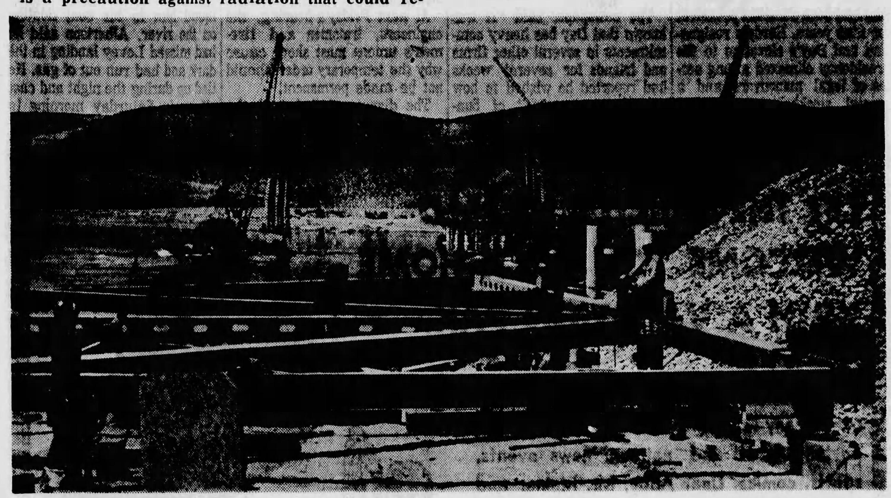
A workman pitched a hot rivet to the catcher as they assembled a portion of the Vernita Bridge superstructure. A completed section was being
