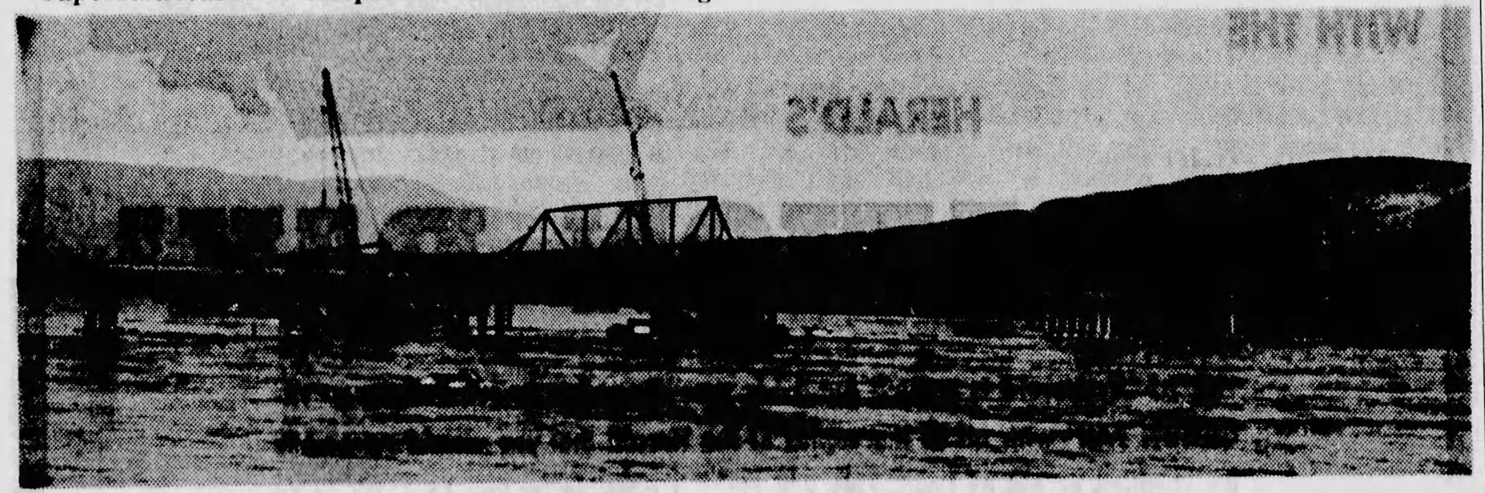
A section of superstructure was lifted into place on the Vernita Bridge and workmen predict the bridge will be completed by the end of August. The \$1.4-million structure will span the Colum-
